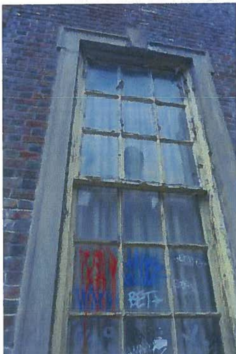
1918-20 Sansom Street, detail of front window and surrounding masonry (August 2015)
