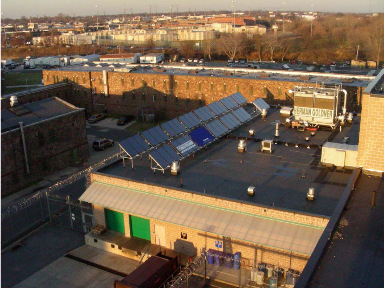
Completed Solar Panel Installation, top of RCF Gym Roof, December 4, 2008
