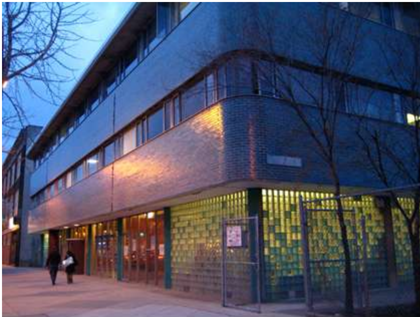
Figure 19: Glass block wall mosaic at the building's northeast corner; note the building's distinctive interior light/nighttime glow
