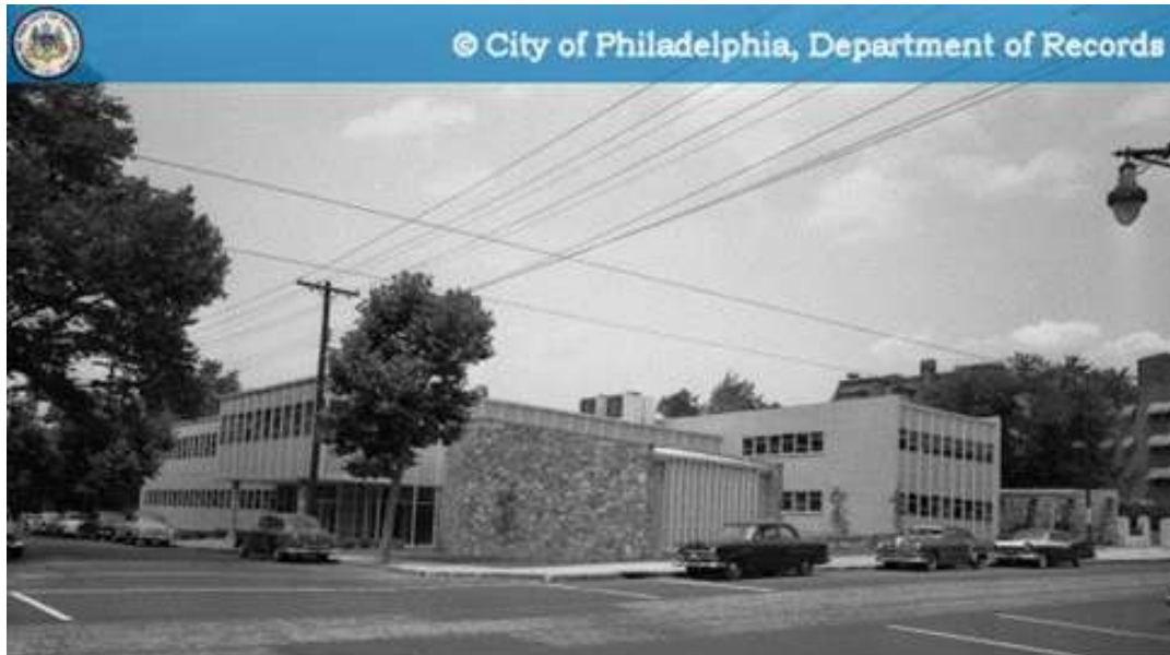
Figure 14B: District Health Center 3 newly completed, June 30, 1960 (PhillyHistory.org, Philadelphia Department of Records)
