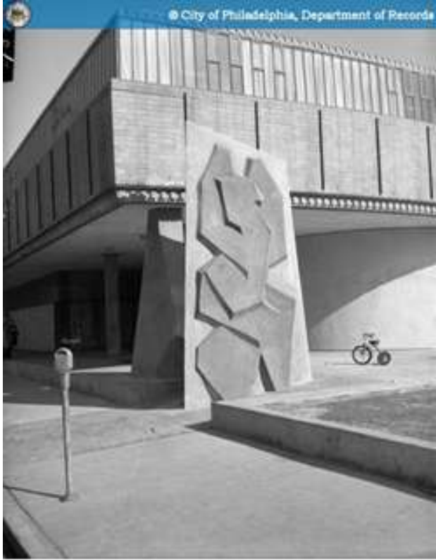
Figure 15A: District Health Center 6, 415 W. Girard Avenue (demolished; PhillyHistory.org, Philadelphia Department of Records)
