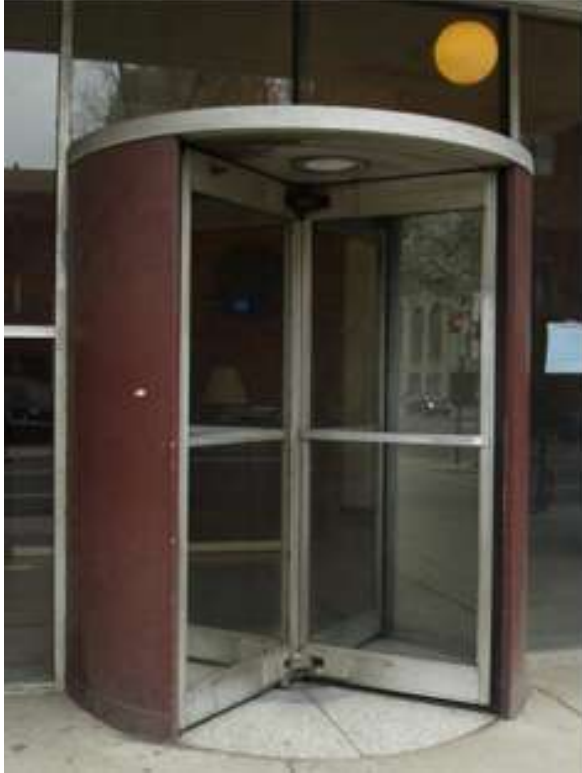
Figure 8: Revolving door at Broad Street entrance (east elevation)
