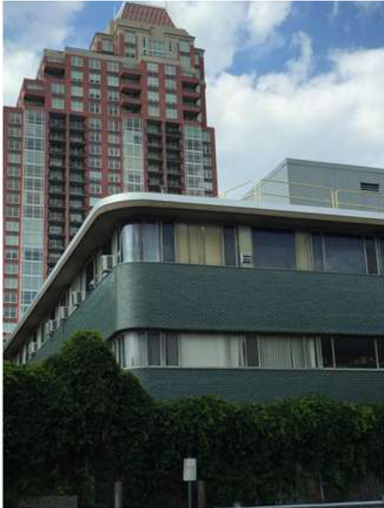
Figure 12: Rounded corners with curved masonry and windows, looking south. Soffit extends a canopy, finished with aluminum.
