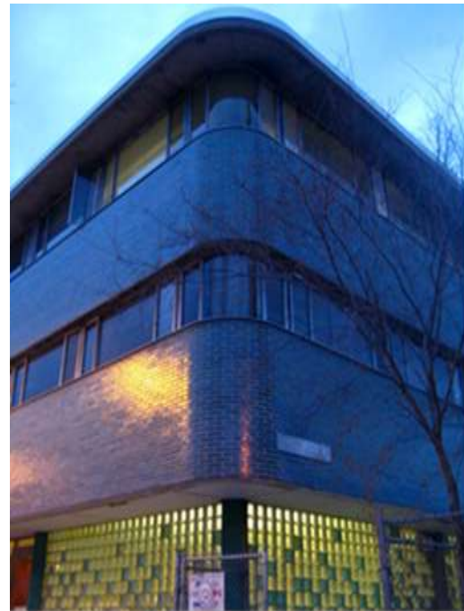
Figures 2A, 2B: Chamfered corner showing rounded masonry from ground level
