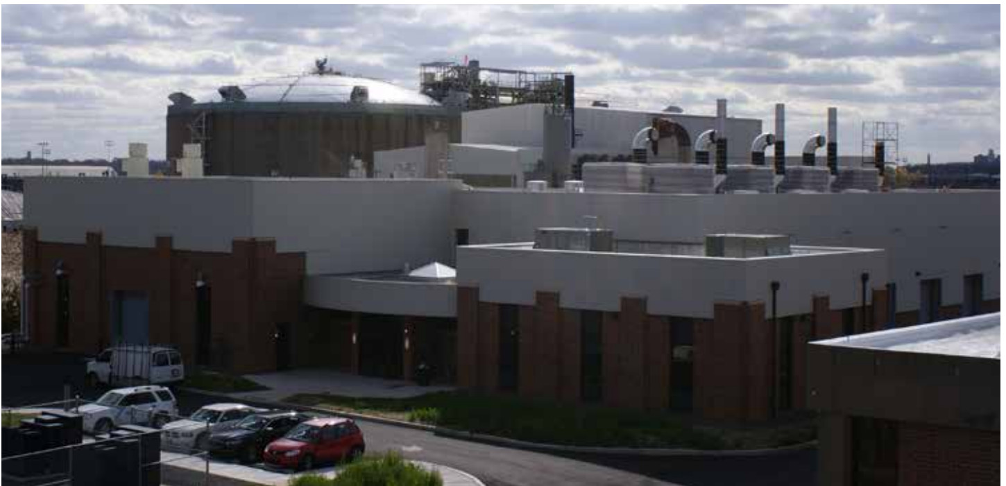
The Northeast Water Pollution Control Plant biogas cogeneration facility.
