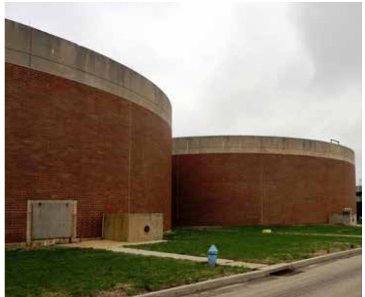
The anaerobic digesters at work.
