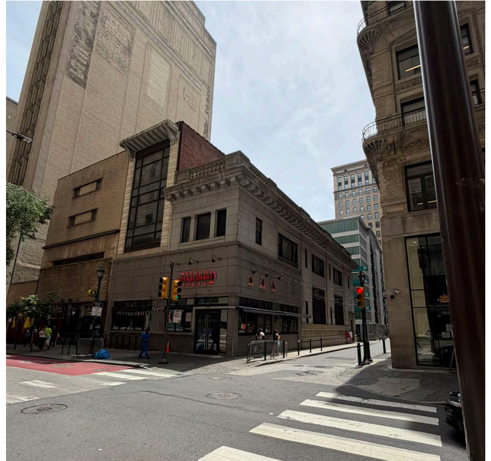
1318-1324 - Facades to the West
