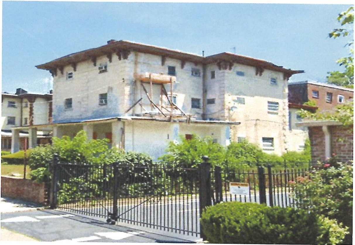
Photo # 5: showing removal of the vegetation and patching the wall.
