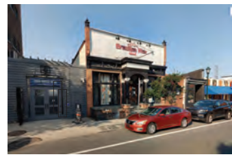
SOUTH WEST VIEW TO FRONT
