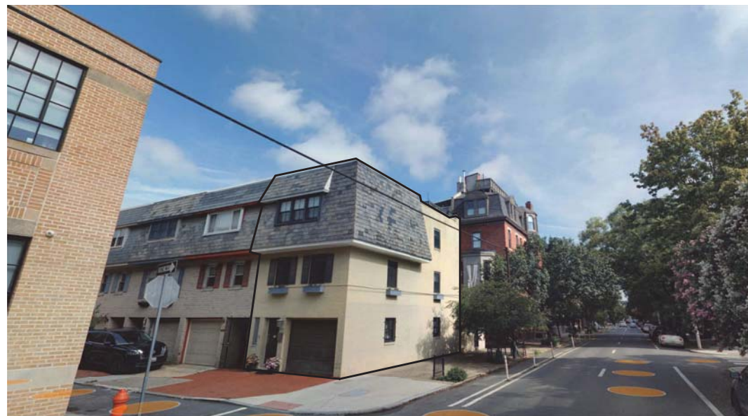
VIEW LOOKING NORTHWEST ON 22ND STREET
