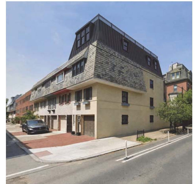
VIEW LOOKING WEST ON 22nd STREET
