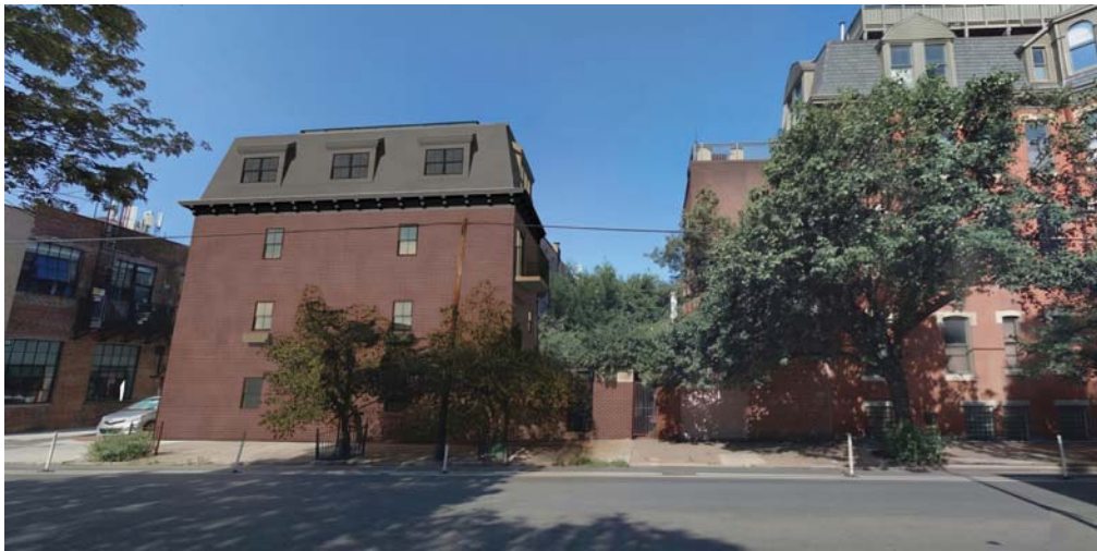
VIEW LOOKING WEST ON 22nd STREET
