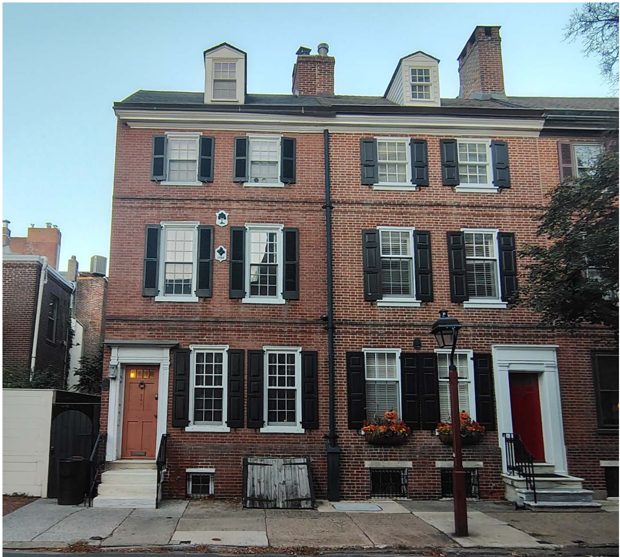
Figure 2: 240 S 7 th St Primary Façade.
