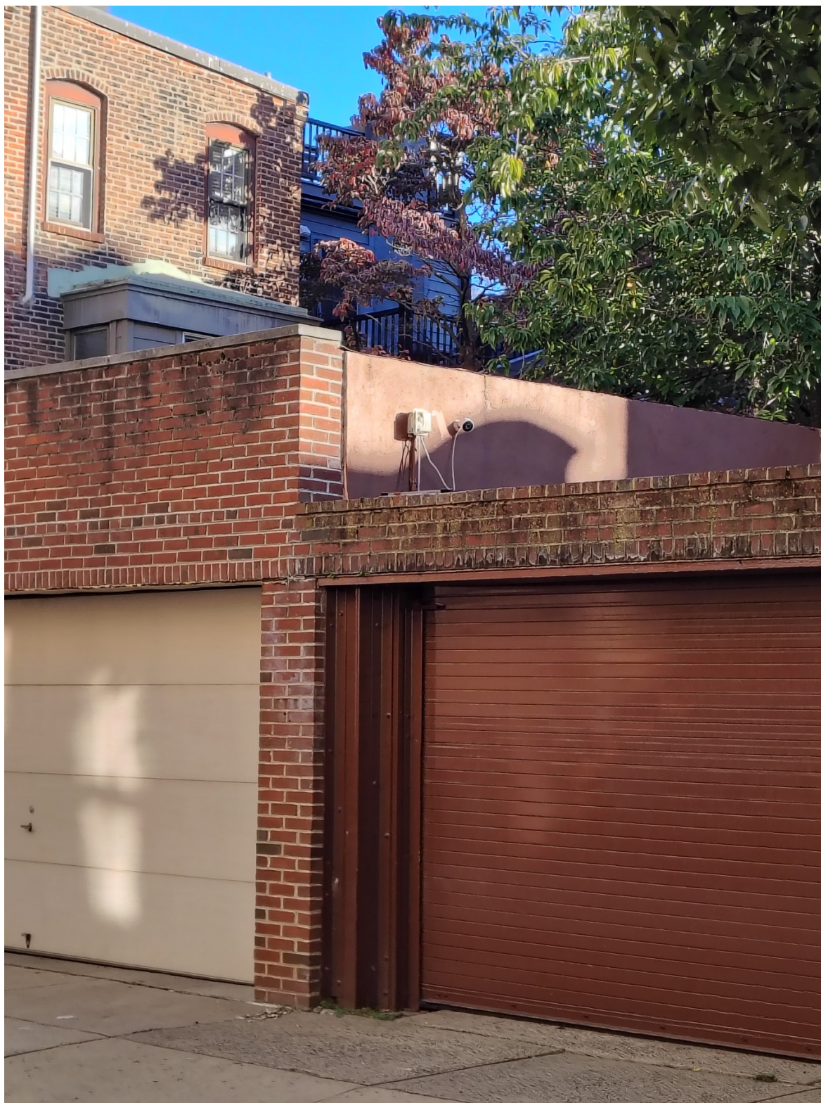
Figure 4: 700 Block of Manning St. Looking towards the rear of 240 S 7 th St. 2 nd & 3 rd Story Decks Visible in Image
