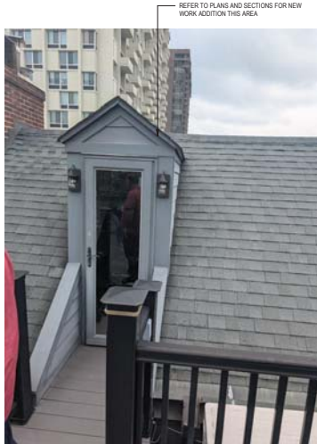
EXISTING REAR WALL AT 4TH FLOOR ROOF DECK
