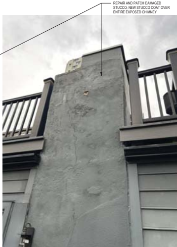
EXISTING REAR WALL AT 3RD FLOOR ROOF DECK, INCLUDING EXISTING CHIMNEY
