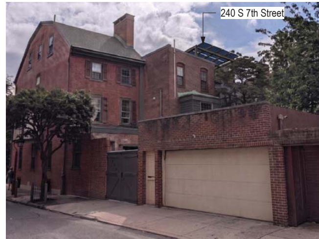
B View looking Southeast from Manning Street
