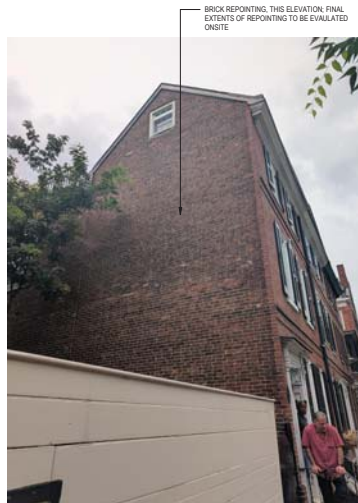
EXISTING SOUTH ELEVATION (PARTIAL)
