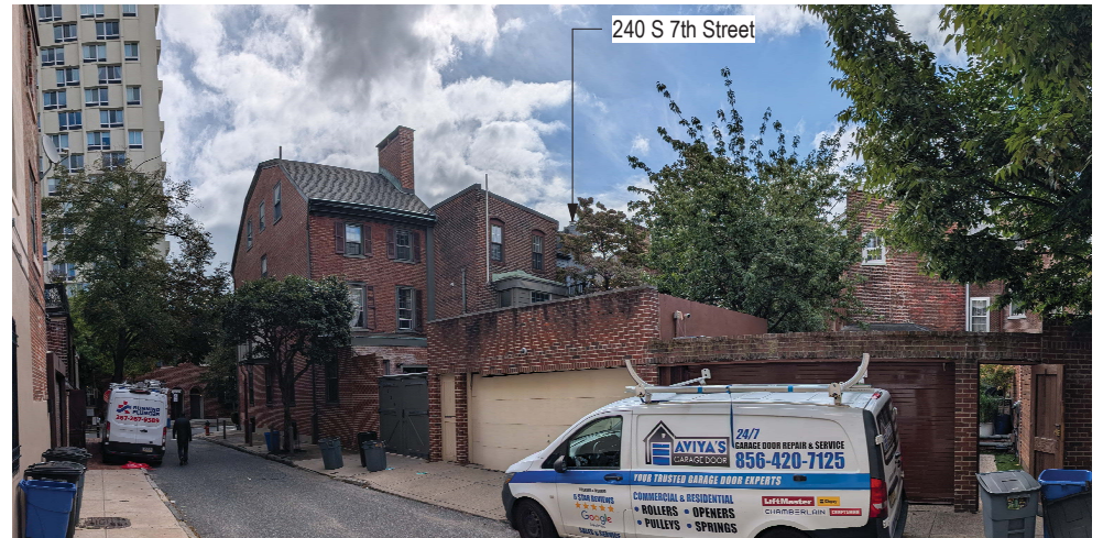
B View looking Southeast from Manning Street
