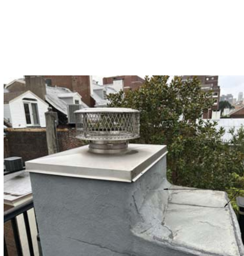
EXISTING TOP OF CHIMNEY AT REAR WALL
