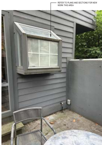
EXISTING REAR WALL AT 1ST FLOOR, LOOKING EAST
