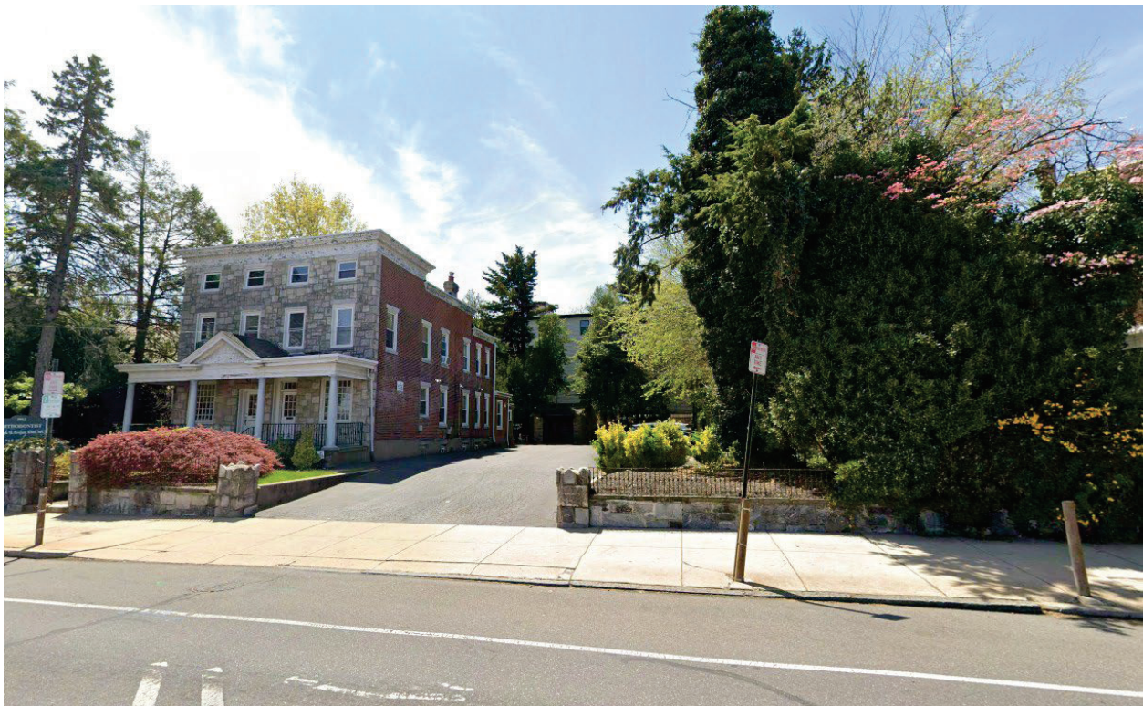
5914 Ridge Ave Philadelphia Historical Commission October/November 2026
