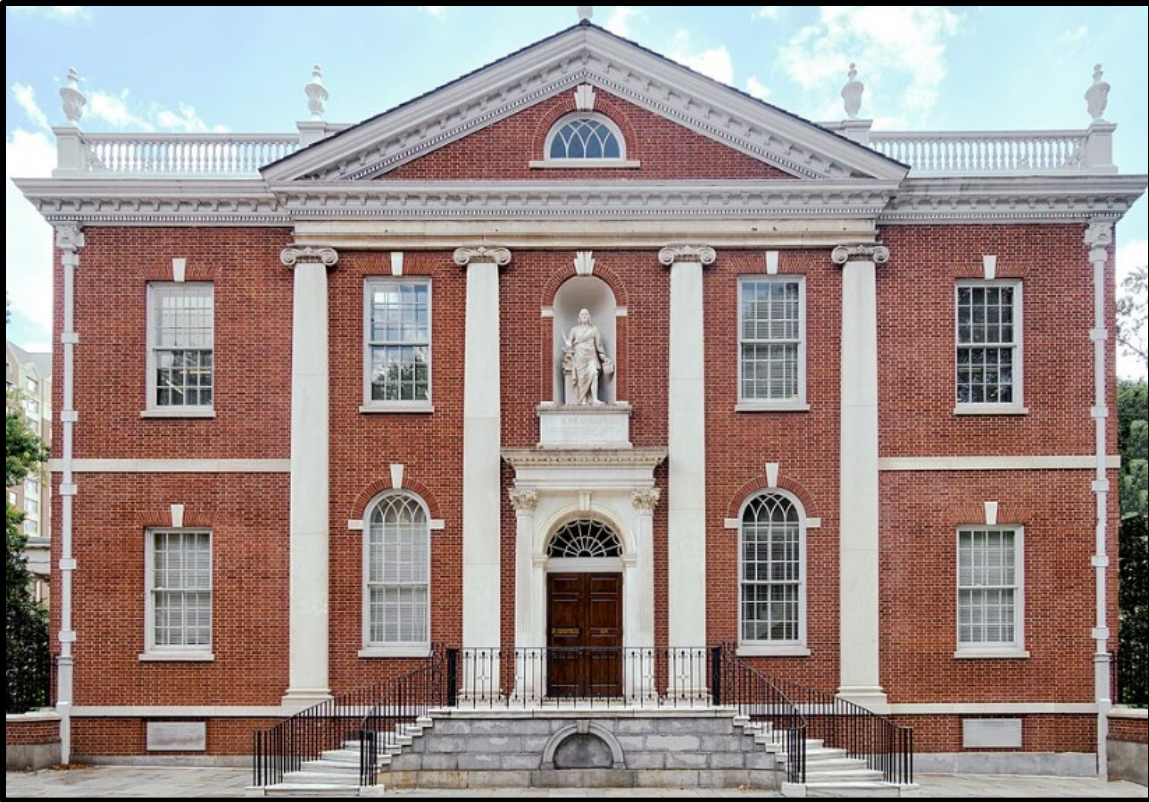
Figure 25. Top: The primary (east) and side (south) elevations of the First Pennsylvania Banking and Trust Company Building in ca.1950-60. Source: Phillyhistory.org. Figure 26. Bottom: The primary (west) elevation of the American Philosophical Society's Library Hall, a replica of the original Library Company of Philadelphia. Source: Eric Kilby.
