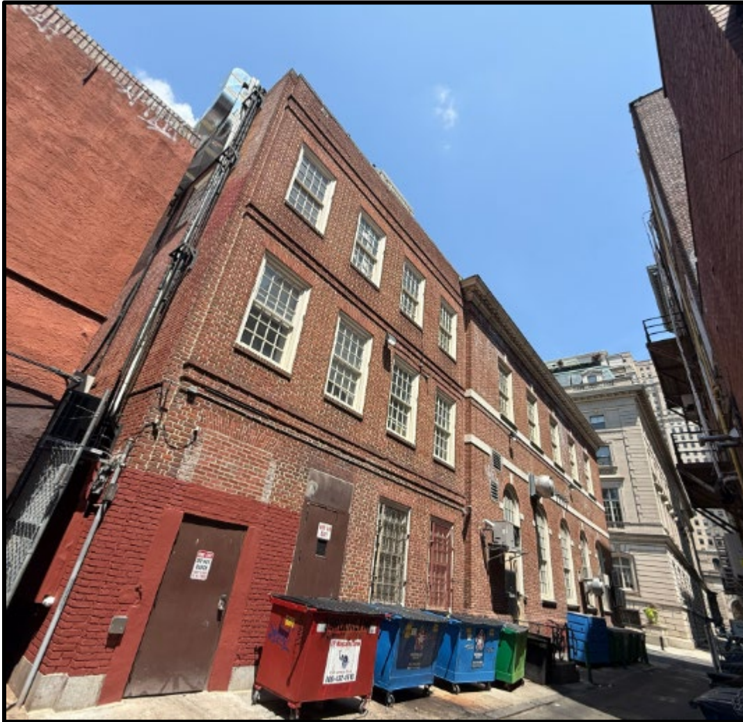
Figure 9. The side (south) elevation of the rear section and the main block. Source: Keeping Society of Philadelphia, 2026.
