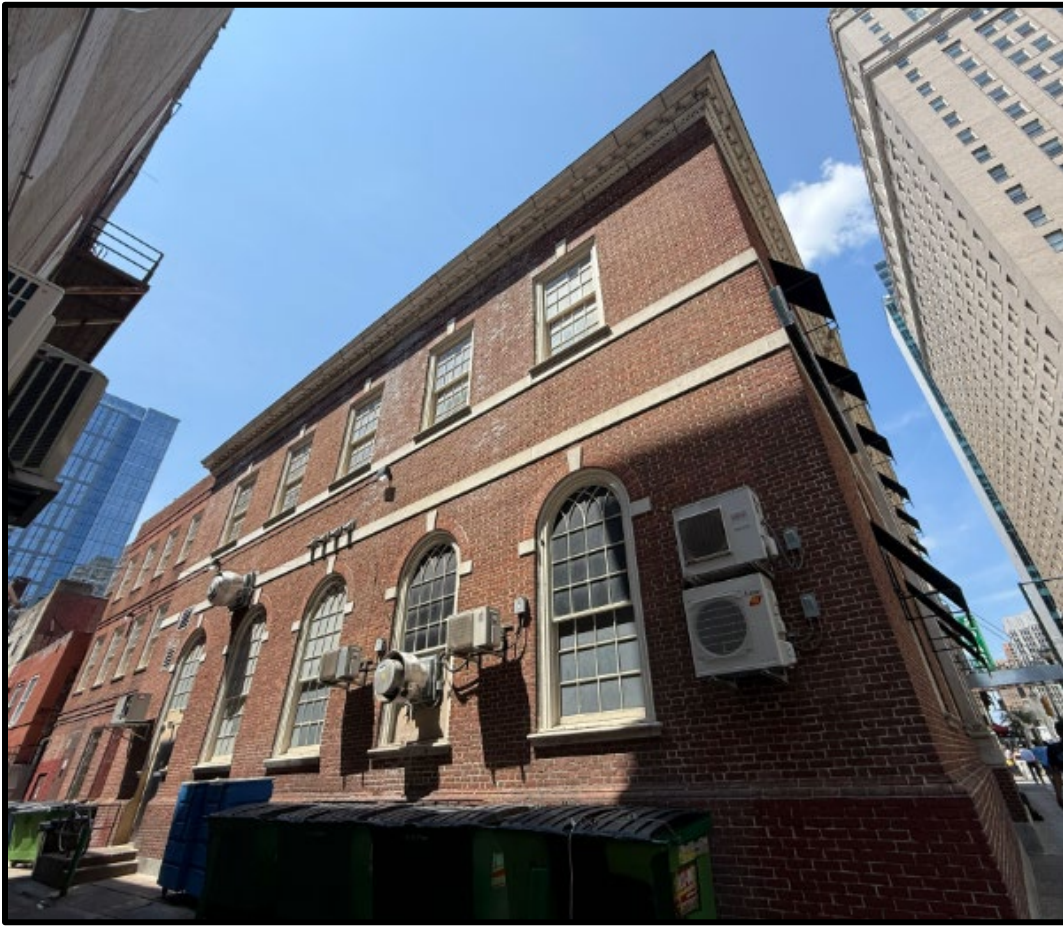
Figure 10. The side (south) elevation of the rear section and the main block. Source: Keeping Society of Philadelphia, 2026.
