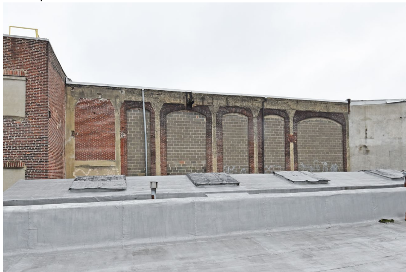
Figure 3: North elevation of the Blacksmith Shop at 121-31 E. Willey Street, looking south. In the foreground is the roof of the one-story Car Shop.
