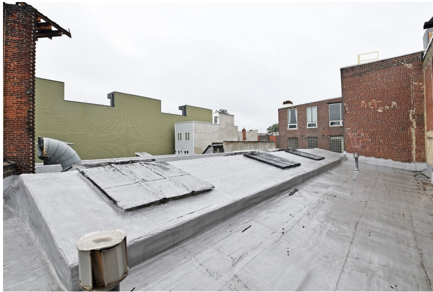
Figure 4: Roof of the one-story Car Shop at 121-31 E. Wildey Street, looking northeast.
