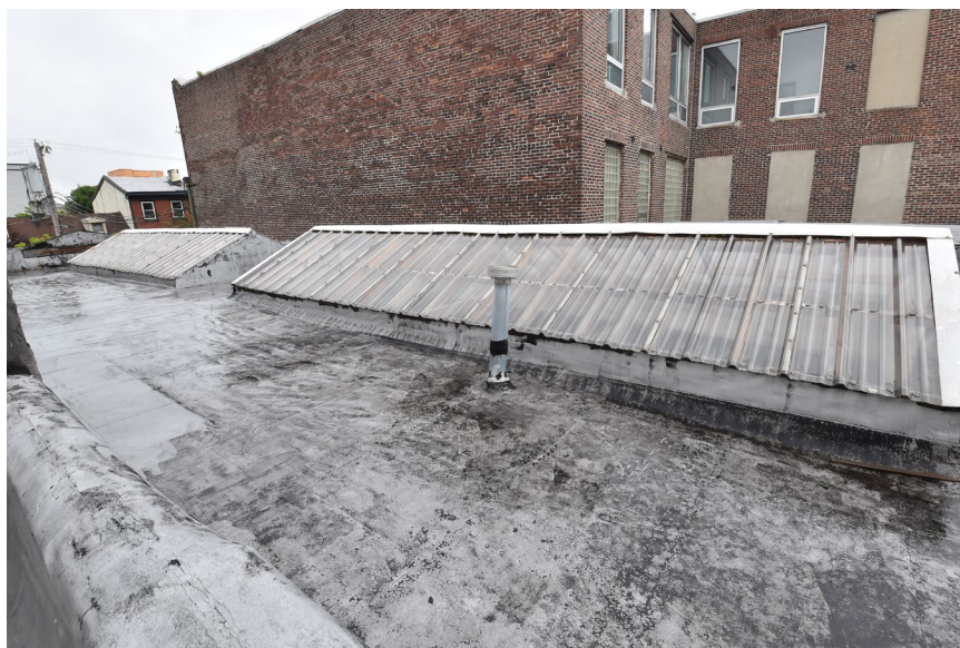
Figure 6: Roof of the Blacksmith Shop at 1108-10 Shackamaxon Street, looking southeast.
