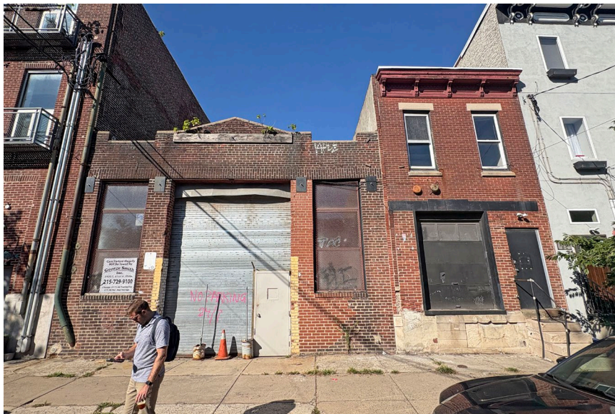
Figure 5: East elevations of the Hindley Gear Company Machine Shop (left) and Storehouse (right) at 1108-10 Shackamaxon Street.
