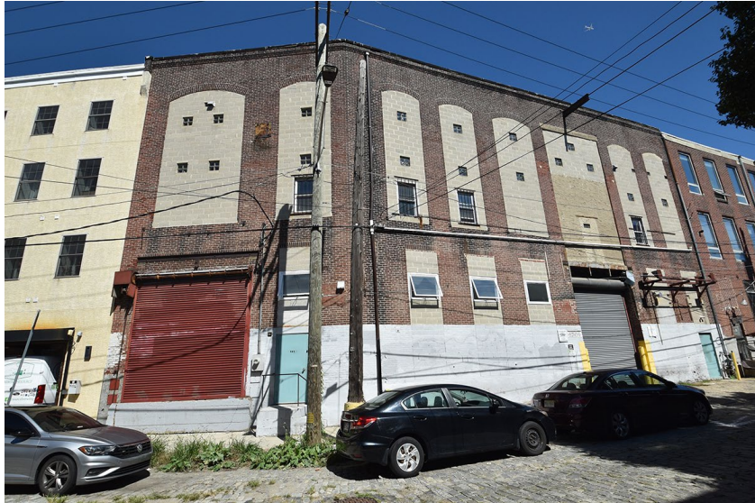
Figure 2: South elevation of the Blacksmith Shop at 121-31 E. Willey Street, looking north.
