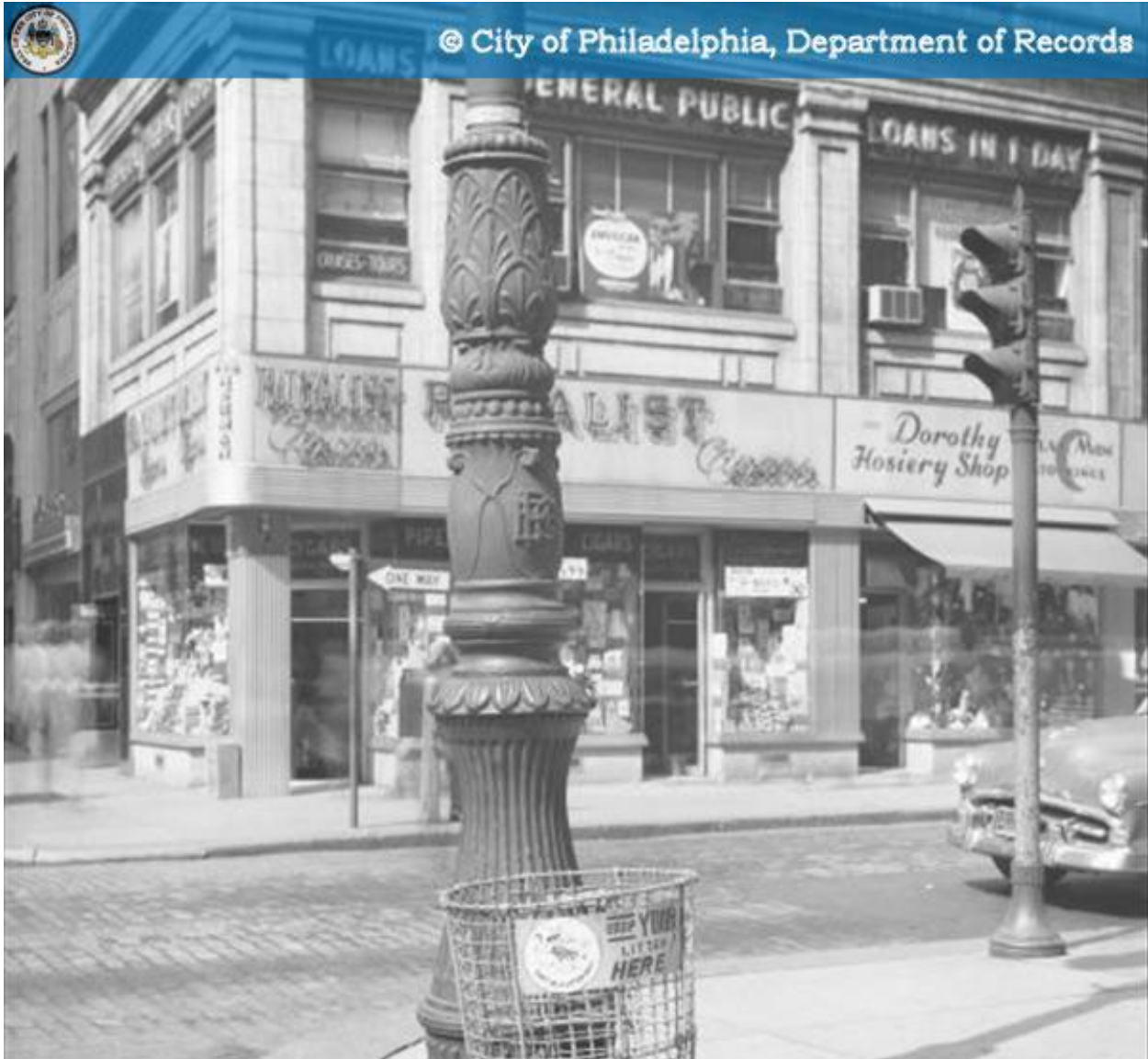
Figure 5: Philadelphia Department of Records photograph, September 29, 1953 (cropped to focus on building). Note the original tripartite division of windows on the second floor on the south elevation; the mullions aligned with the panel rails below.
