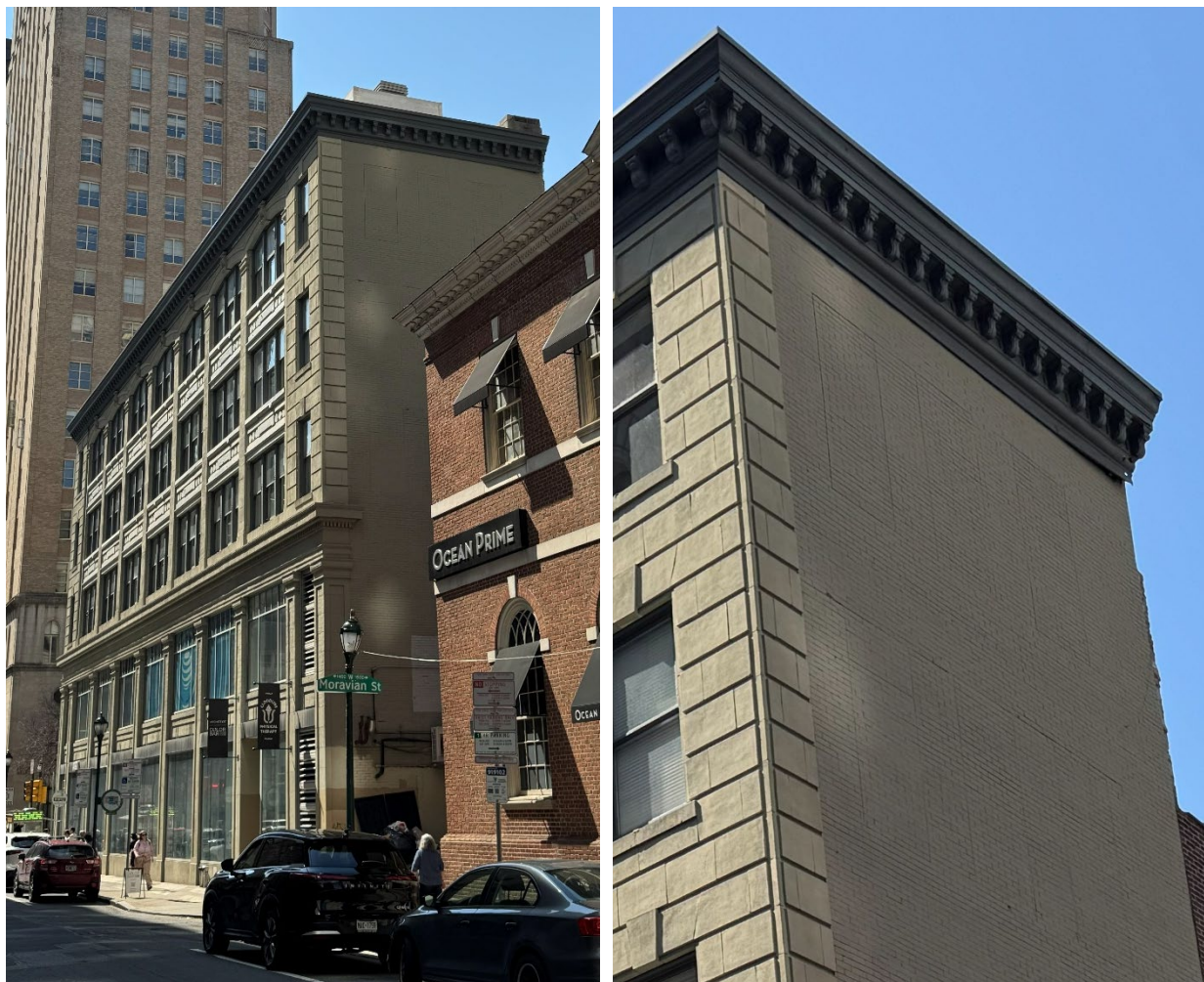
Figure 9a & 9b: Partial view of north elevation (left). Windows at the Moravian Street elevation have been infilled. Ghosts of the old windows are still visible (right). Photos by author, March 26, 2026.
