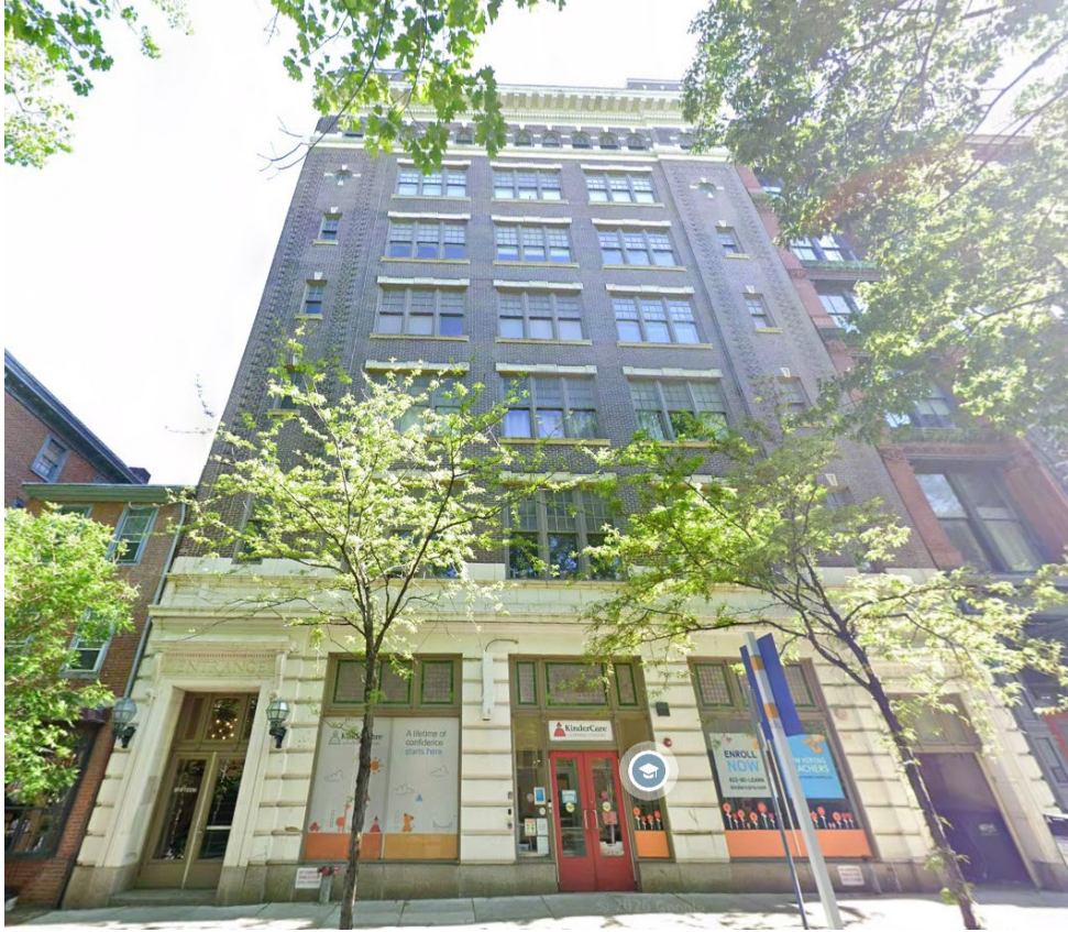
Figure 29: Schmidt Building, 315-19 Arch St., Sauer & Hahn, 1915. Source: Google Maps.
