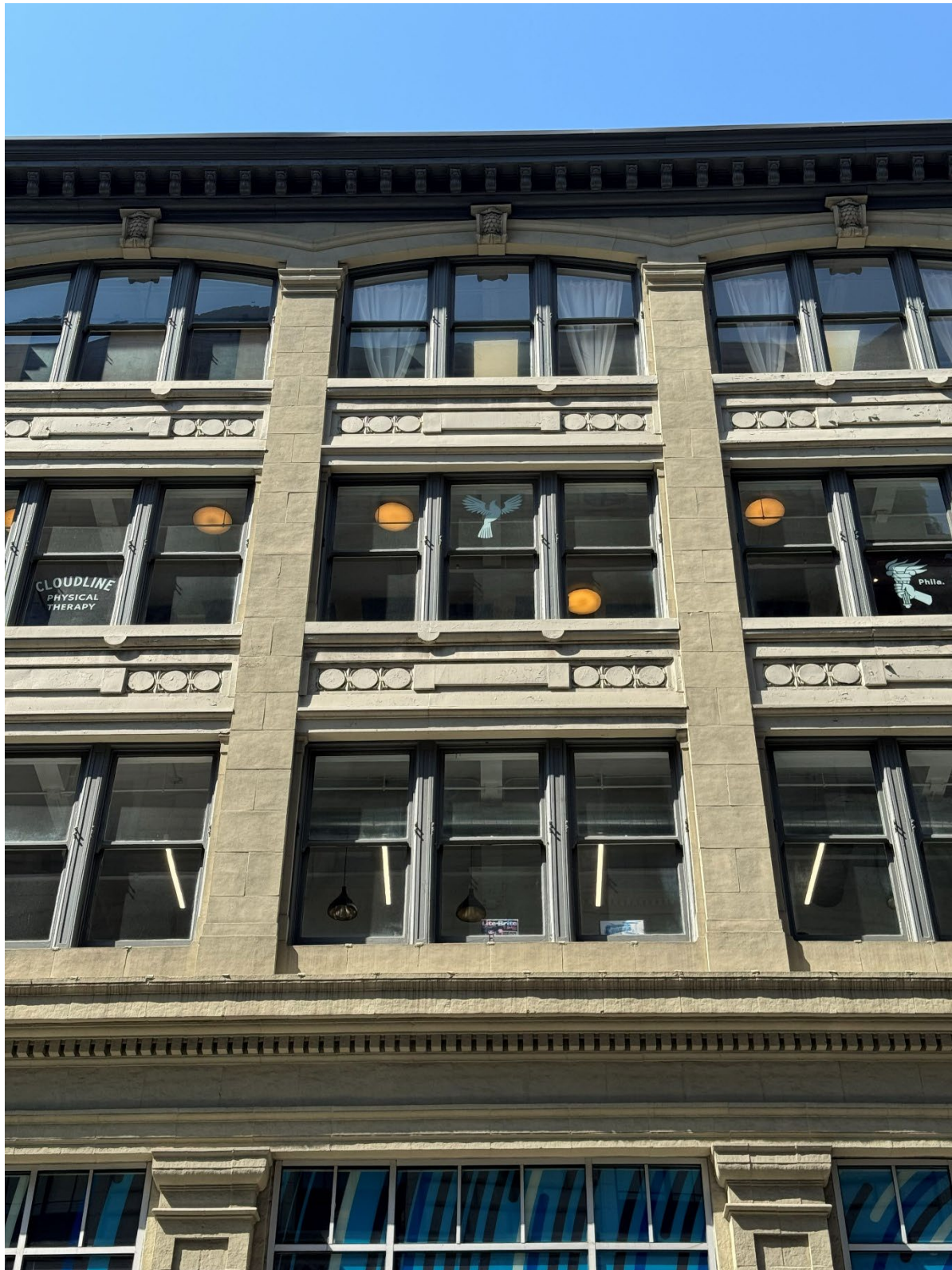
Figure 6: Detail of center bay, upper three stories. Note monumental pilasters vertically linking three stories of window openings, abstracted classical orders, and flattened, simplified ornament. Photo by author, March 26, 2026.
