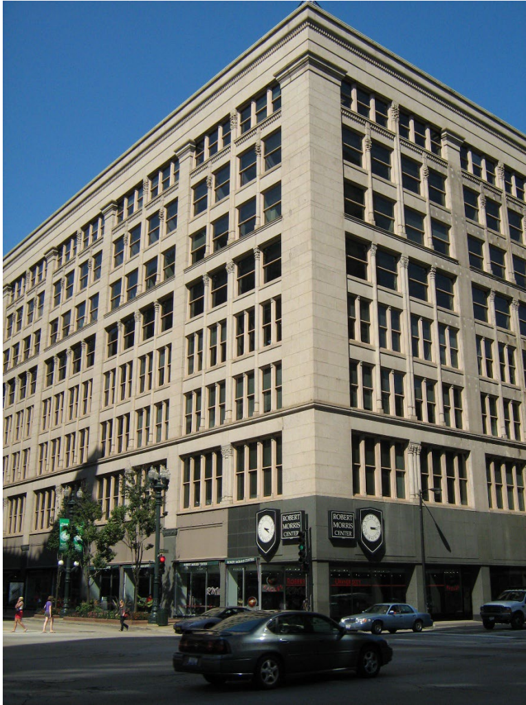
Figure 25: Leiter II Building, William LeBaron Jenney (1891, Chicago, Illinois) Source: Zol87 (on Flickr), Leiter II Building , February 16, 2011, photograph, https://commons.wikimedia.org/w/index.php?curid=13318928 .
