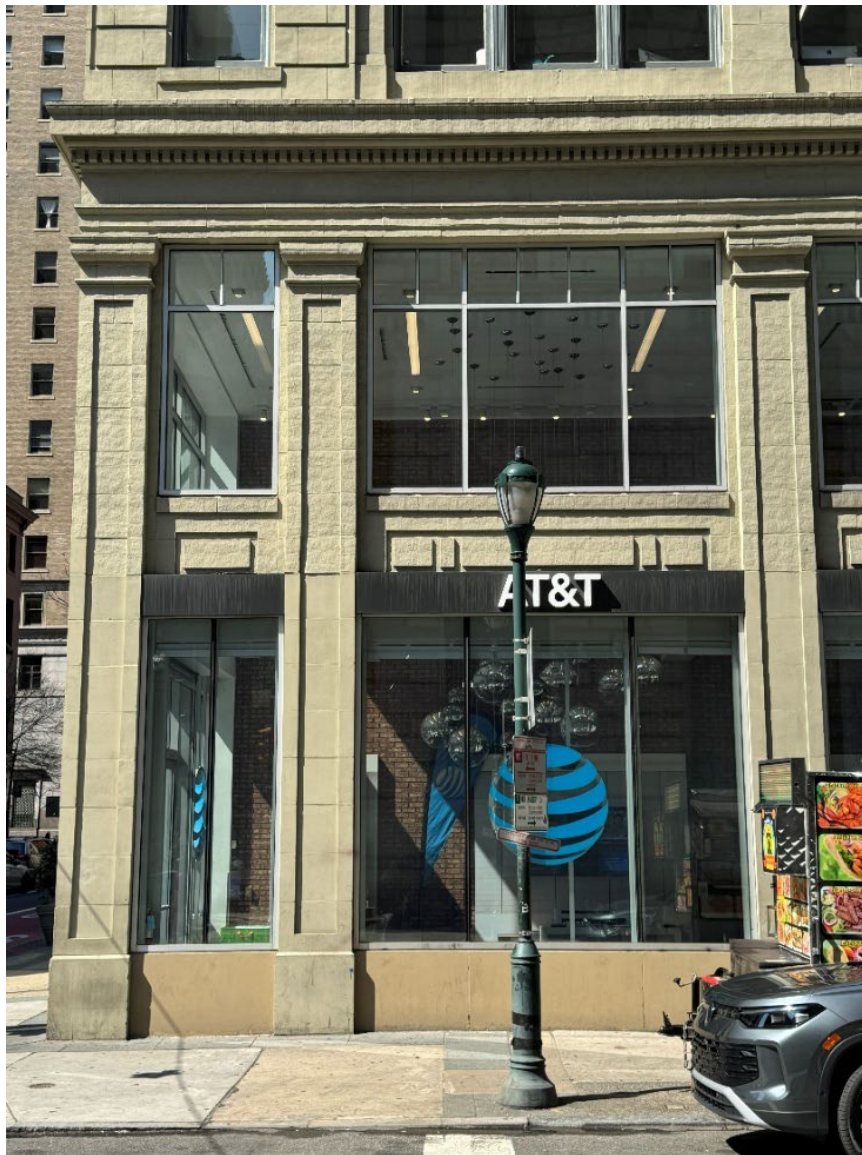
Figure 7: Enlarged view of southernmost bays along east (15th Street) elevation. These replacement storefronts were added during the 2015 renovation of the building; it appears as though some stone on the pilasters was replaced at this time as well. Photo by author, March 26, 2026.
