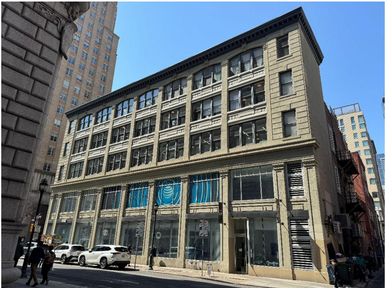
Figure 3: East elevation, 1501 Walnut Street. Note the tripartite division typical of classicism. Here, the bottom two stories and the top three are divided into almost equal halves. Photo by author, March 26, 2026.
