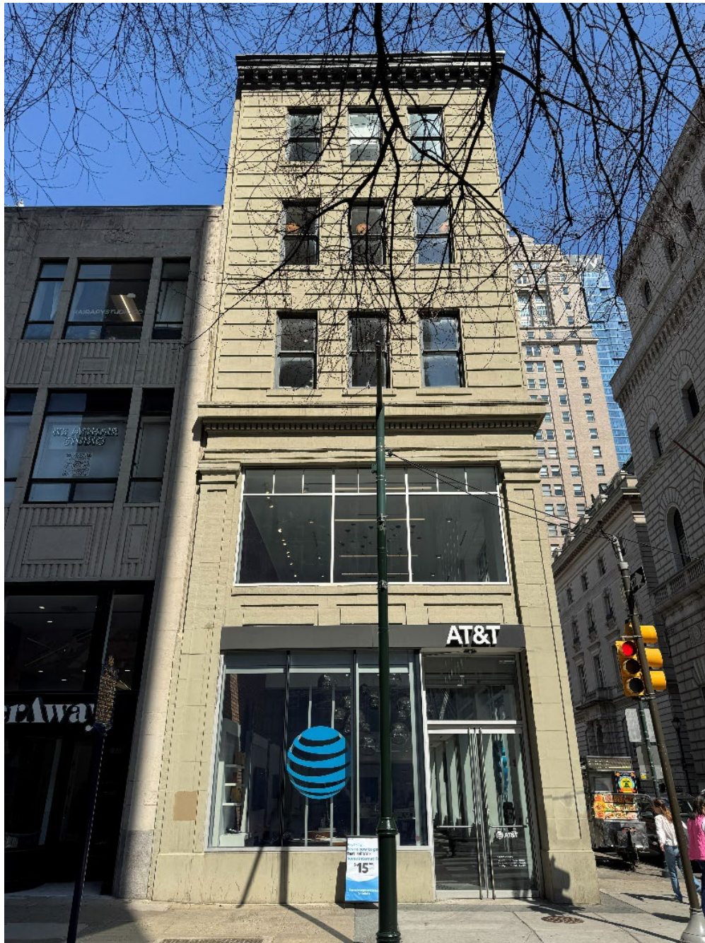
Figure 4: South elevation, along Walnut Street. The lower two stories were substantially altered in 2015, including moving the entrance and installing new storefront. Photo by author, March 26, 2026.
