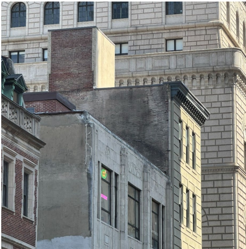
Figure 10: Partial view of west elevation and elevator overrun from further west along Walnut Street. Photo by author, March 26, 2026.
