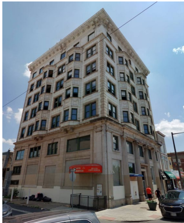
Figure 10: The Ludlow Street elevation seen obliquely from 52 nd Street. Cyclomedia, 2025.
