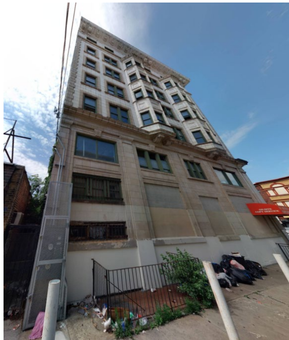
Figure 9: The northeast corner of the Parke Building.
