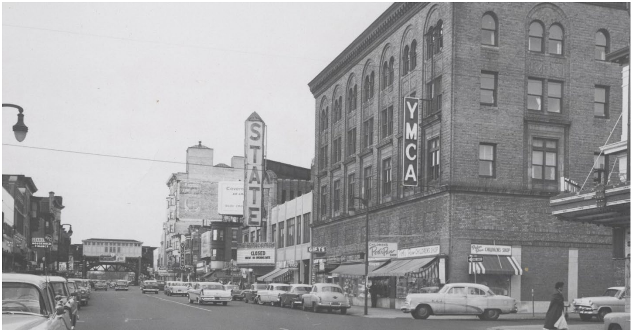
Figure 44: 52 nd Street seen in 1959, before both the State Theatre and the YMCA were demolished. Detail of photograph by Bob Fox, Free Library of Philadelphia Print and Picture Collection.
