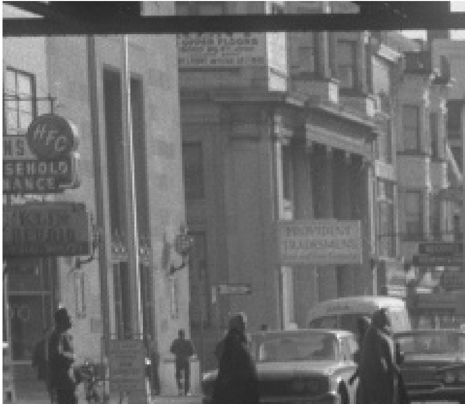
Figure 41: The renovated primary elevation of the Parke Building, with the Philadelphia Saving Fund Society branch bank (built 1926-27) visible in the foreground across Ludlow Street. Detail of 1961 photograph attributed to "Bender," Philadelphia City Archives, Law Department collection.
