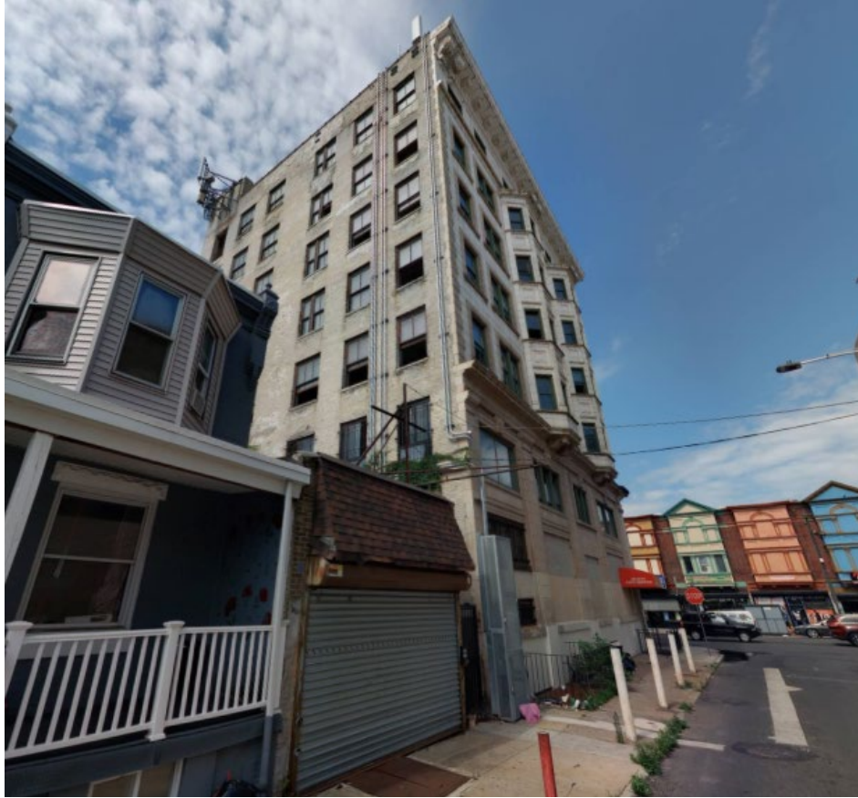
Figure 11: Oblique view of the east elevation, seen from Ludlow Street. Cyclomedia.
