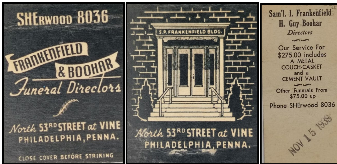
Figure 25. Various views of a matchbook dated 15 November 1939, may show the primary entrance as it appeared in the years after the porch was enlarged. Source: Ebay.
