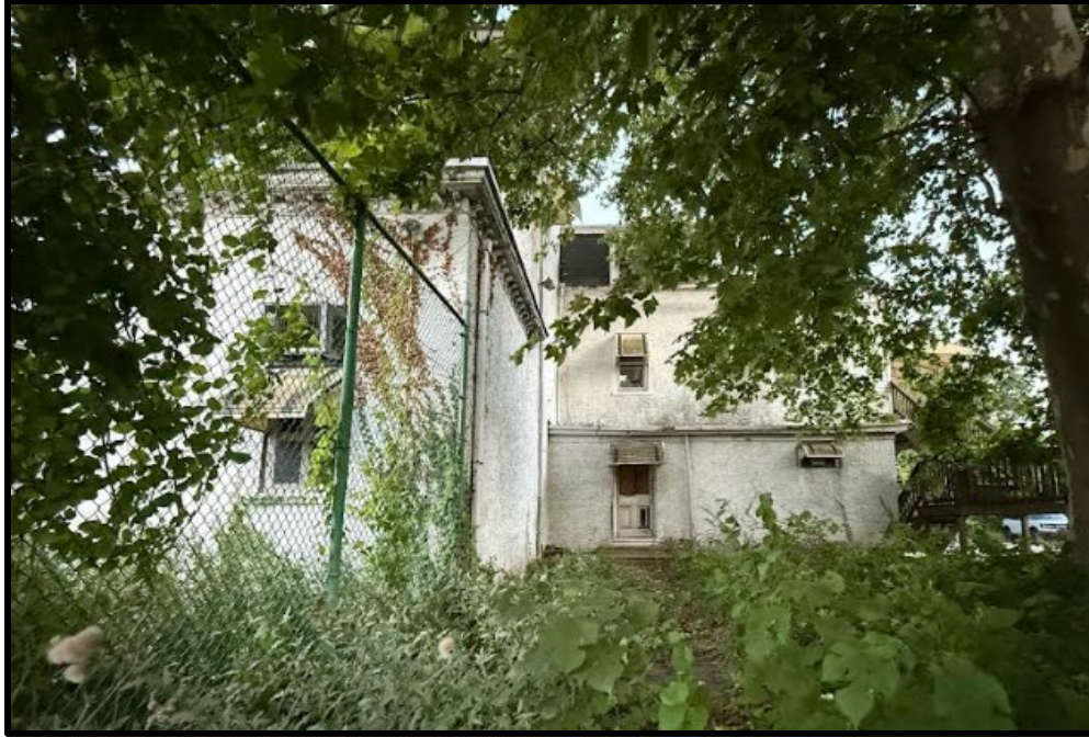
Figure 8. The side (north) elevation of the rear wing and later additions. Source: Keeping Society of Philadelphia, 2026.
