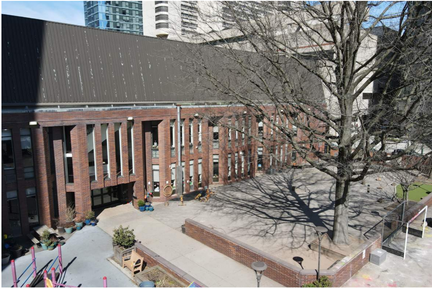
VIEW FROM BACKLOT LOOKING NORTHWEST (ROOF LEVEL)
