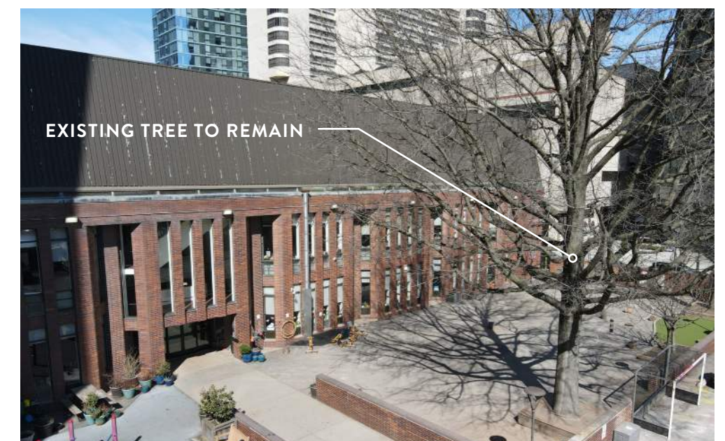
VIEW FROM BACKLOT LOOKING NORTHWEST (ROOF LEVEL)
