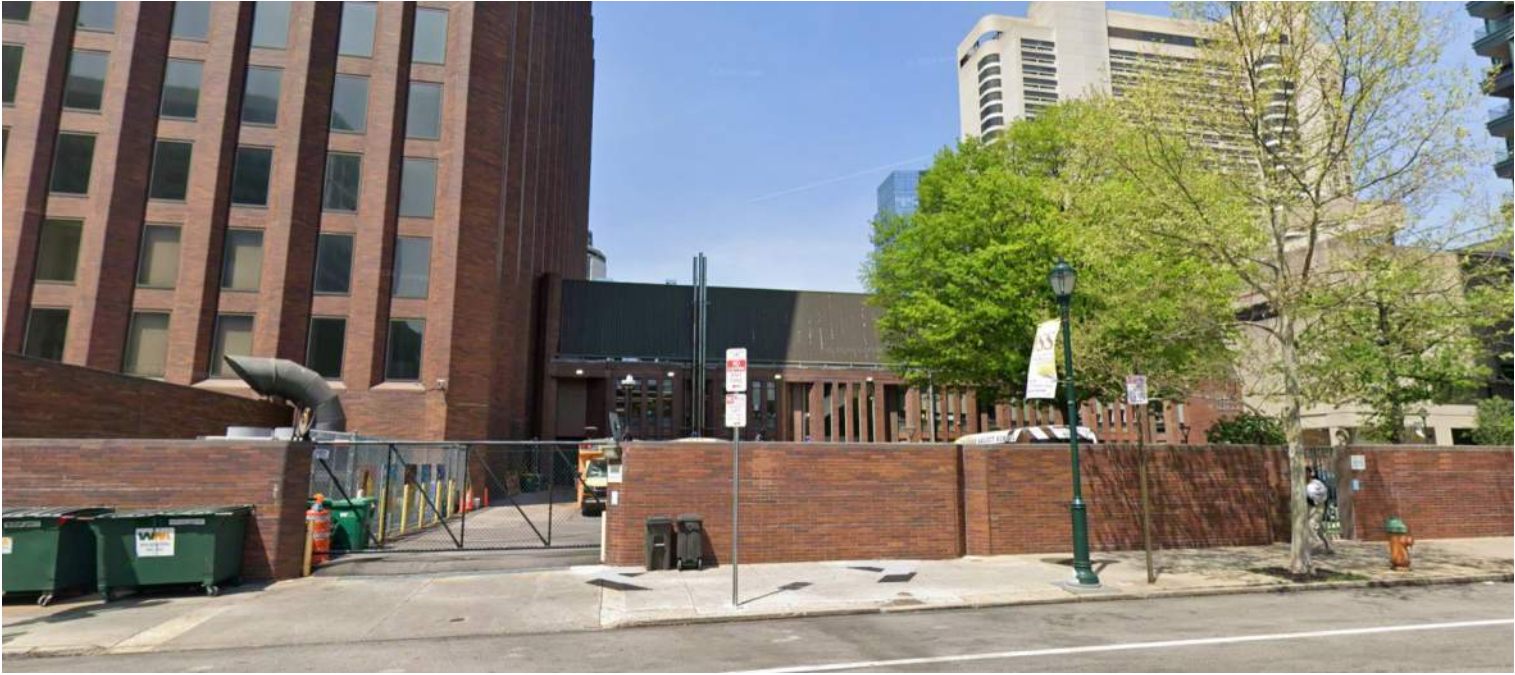
16TH STREET LOOKING WEST
