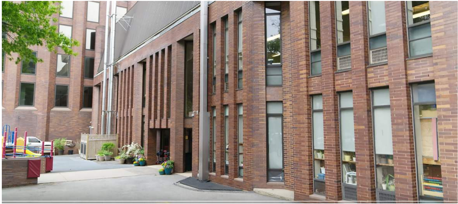
VIEW FROM BACKLOT LOOKING SOUTHWEST TOWARD SCHOOL
