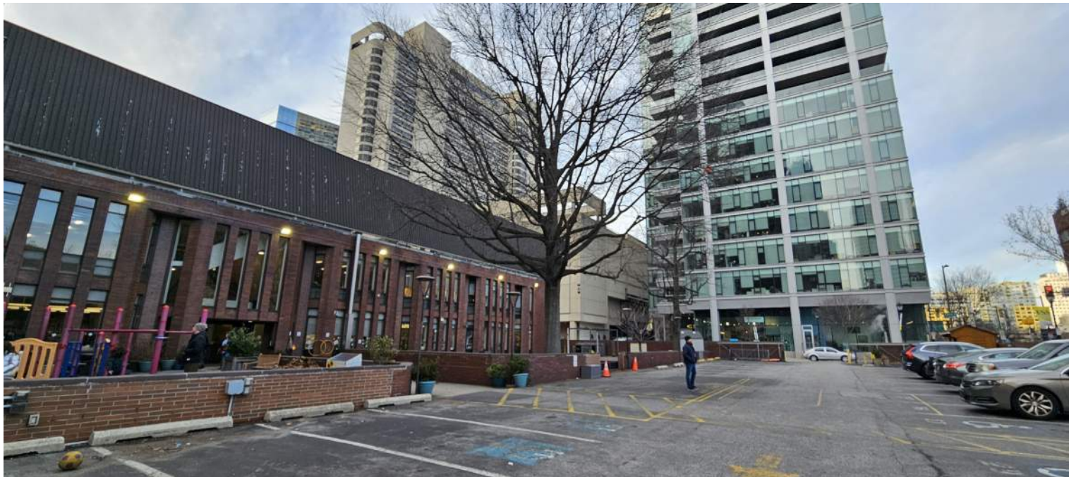
VIEW FROM BACKLOT LOOKING NORTHWEST (STREET LEVEL)
