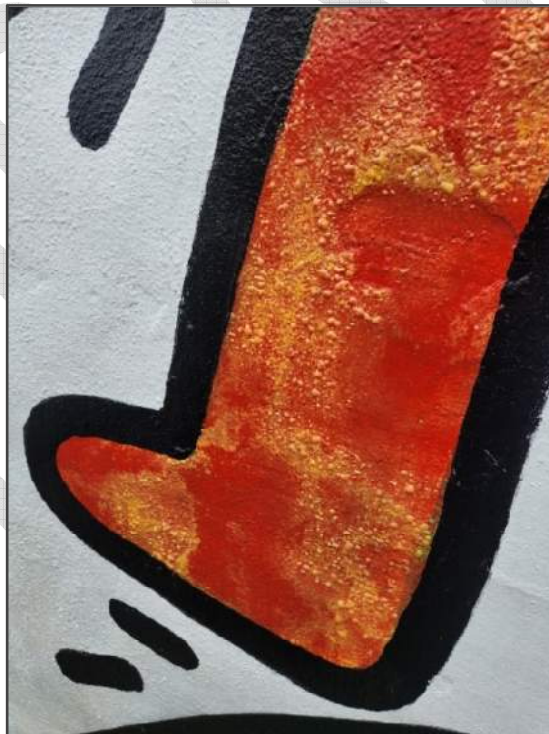
Photo No. 9: Bubbling paint
