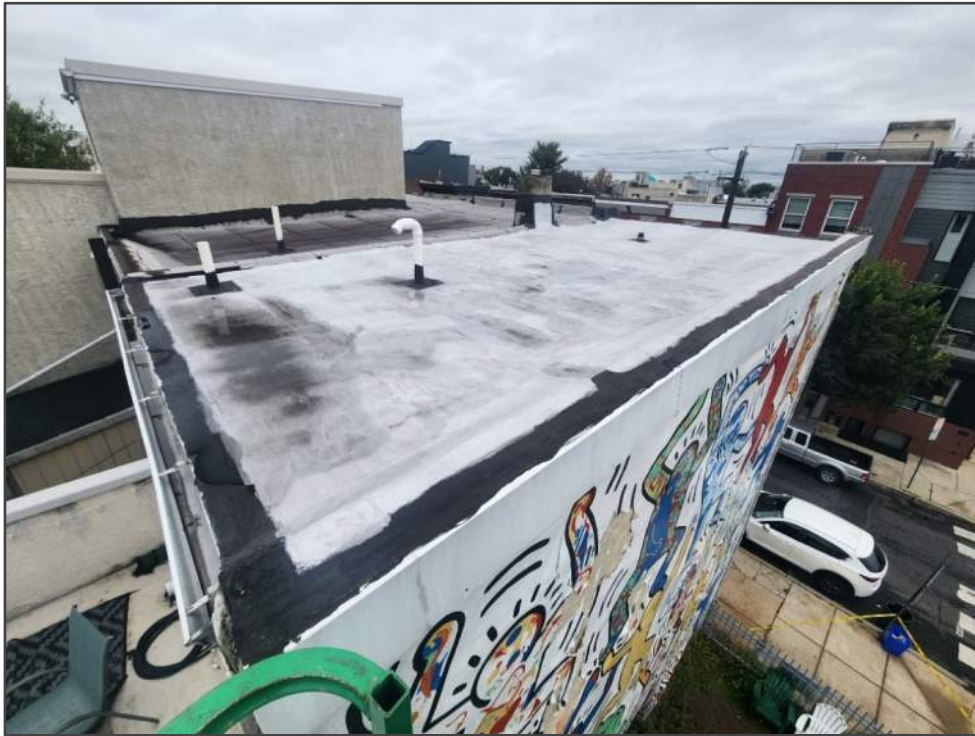
Photo No. 2: Main roof/top of wall condition
