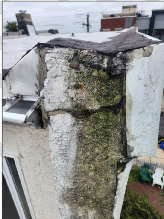
Photo No. 3: Top of 3 rd floor wall condition
