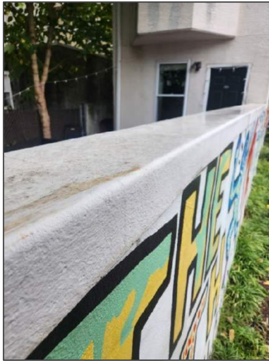
Photo No. 16: Top of site wall condition
