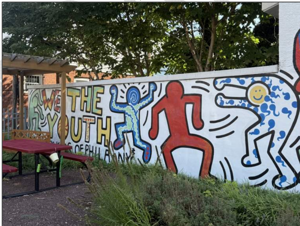
Photo No. 17: Site wall in good condition
