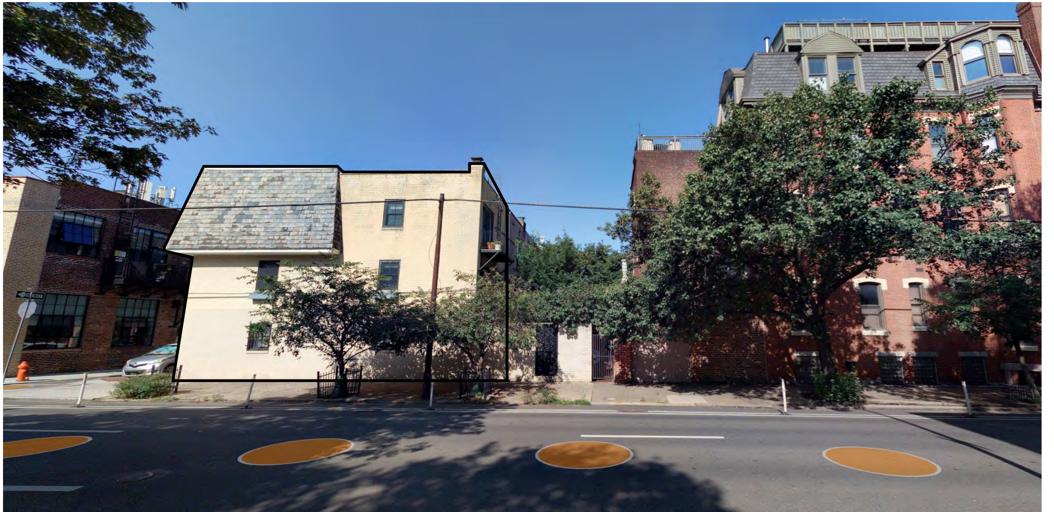
VIEW LOOKING WEST ON 22ND STREET
