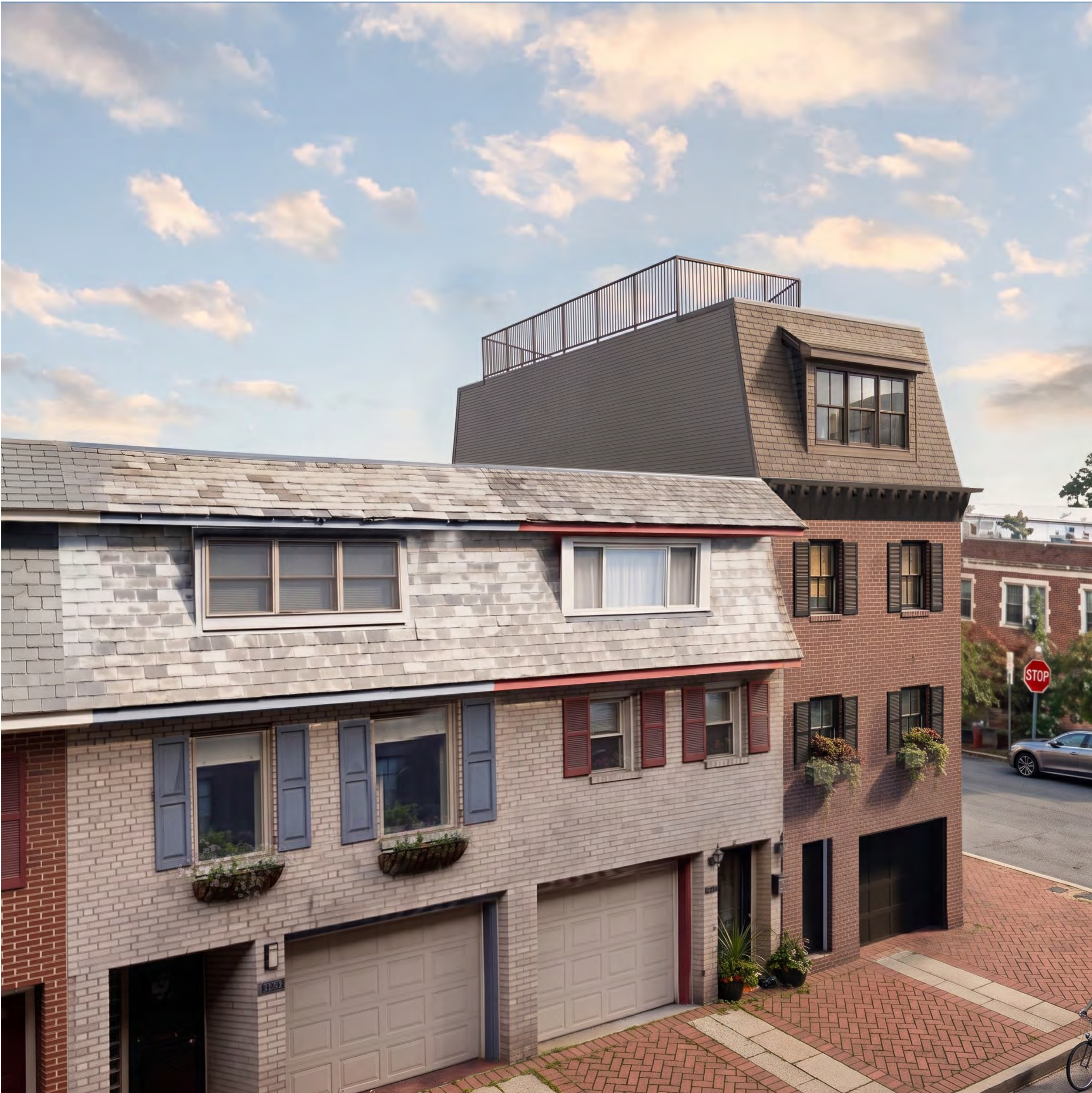
VIEW LOOKING EAST ON PANAMA STREET
