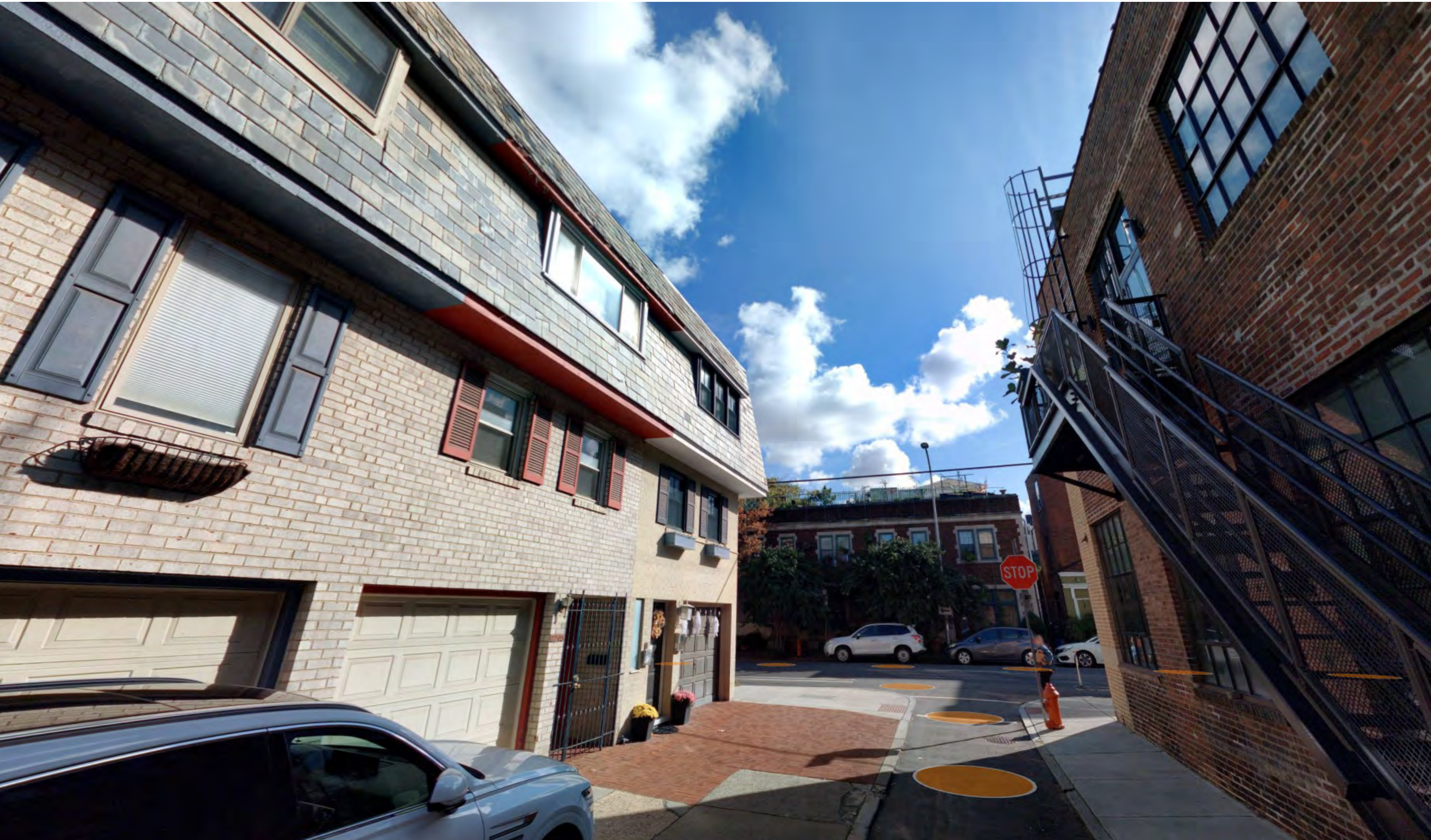
PANAMA STREET LOOKING EAST
