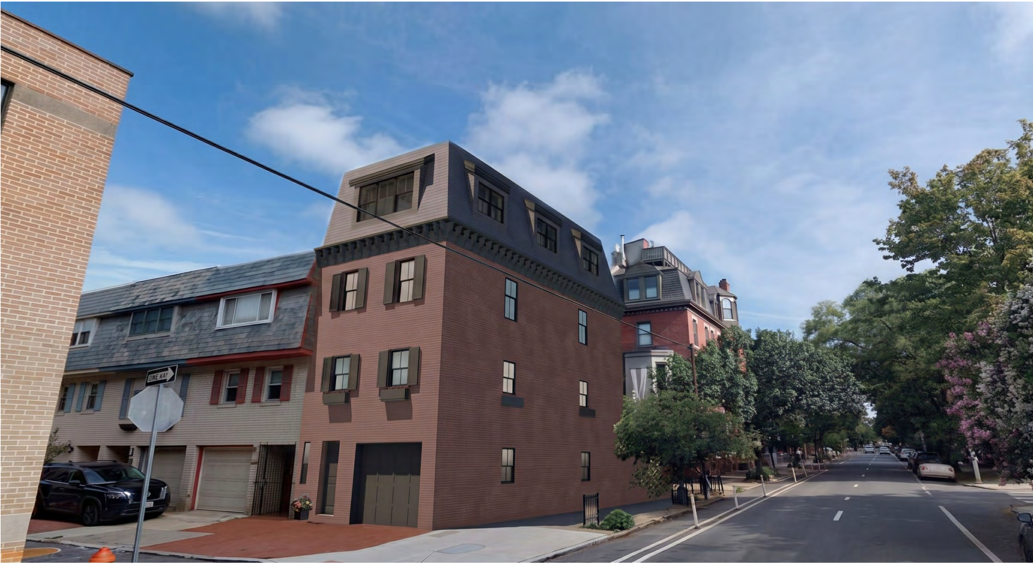
VIEW LOOKING NORTH ON 22nd & PANAMA STREETS
