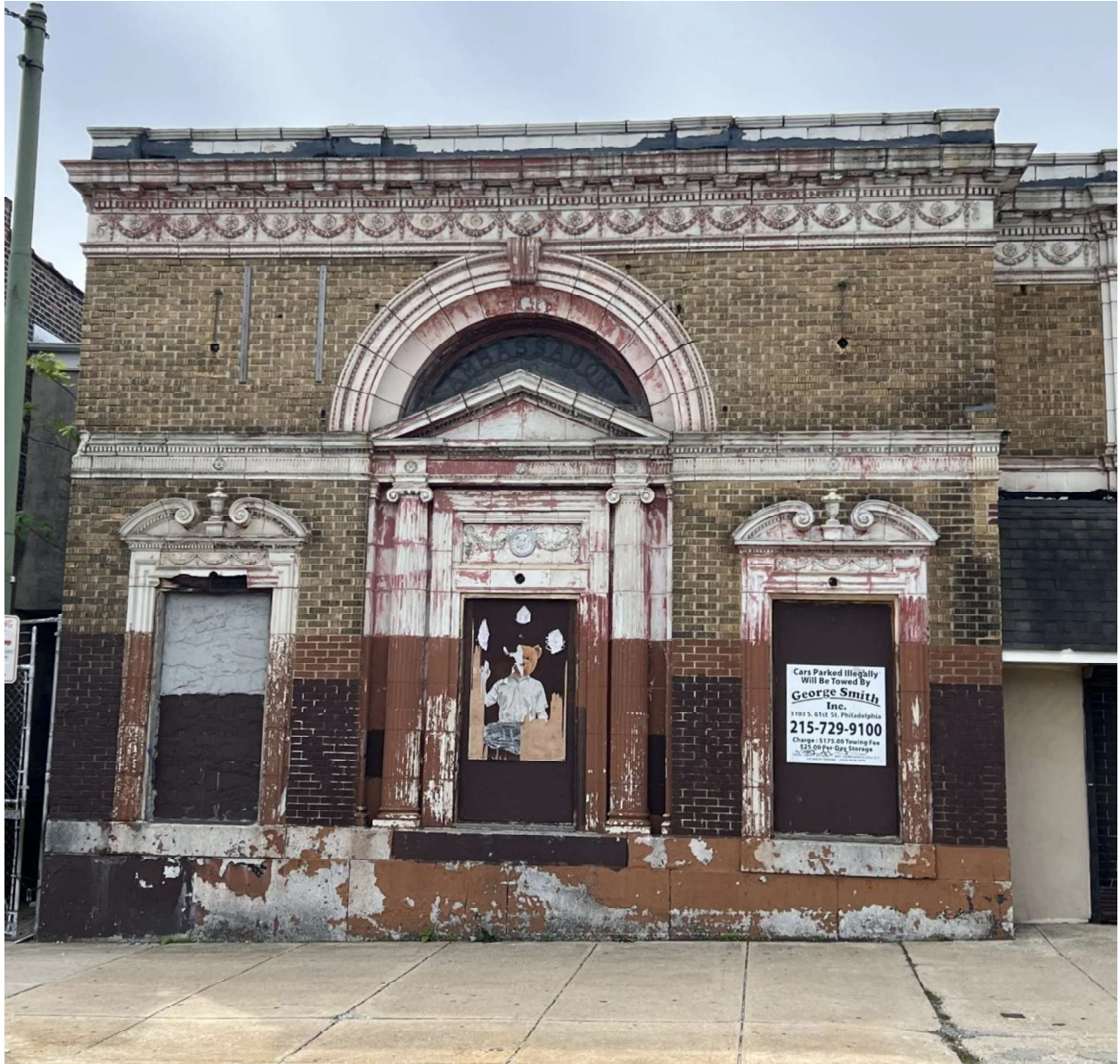
Figure 9: View of the facade's east volume.
