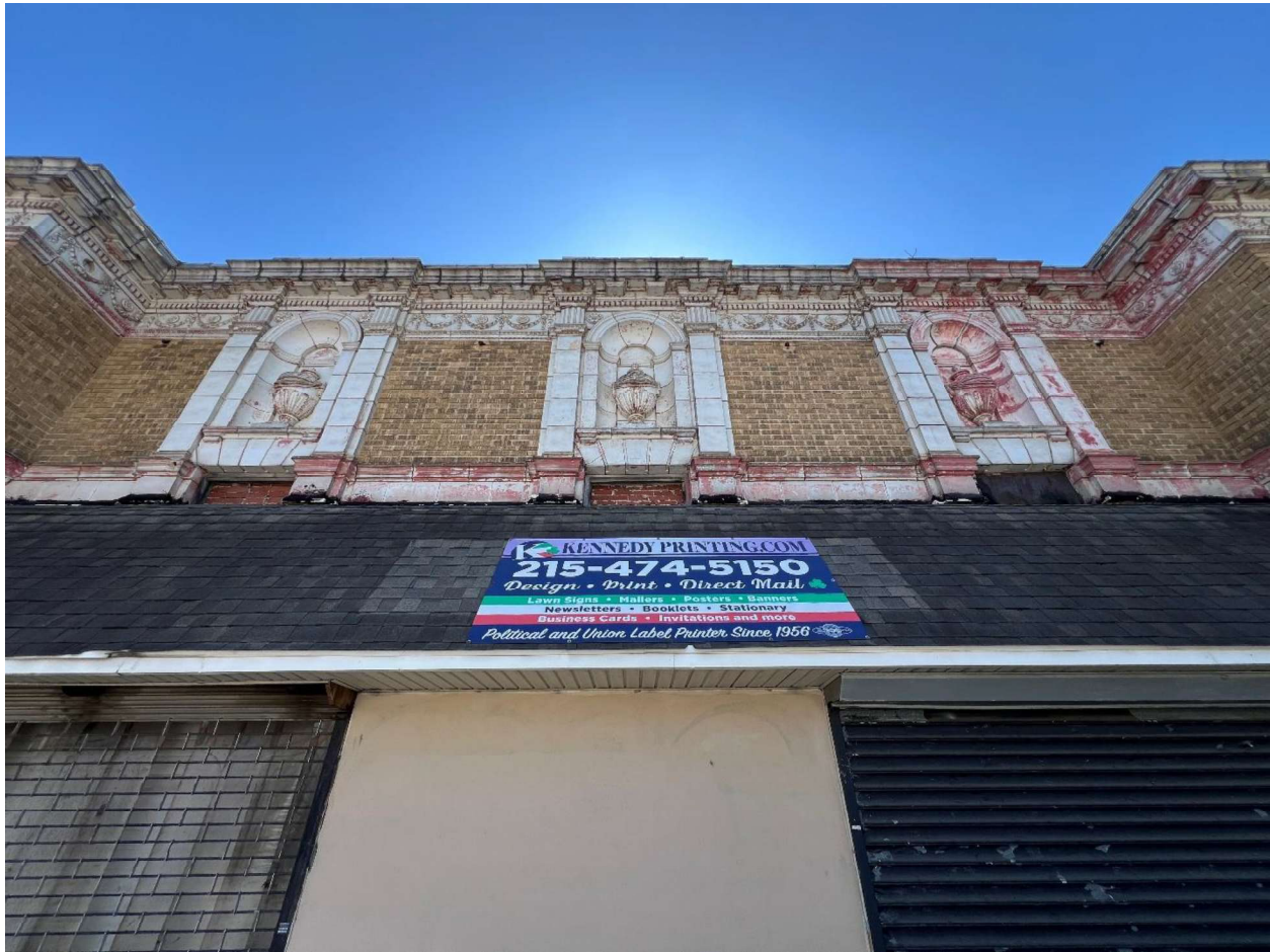
Figure 12: View of the facade's central volume.
