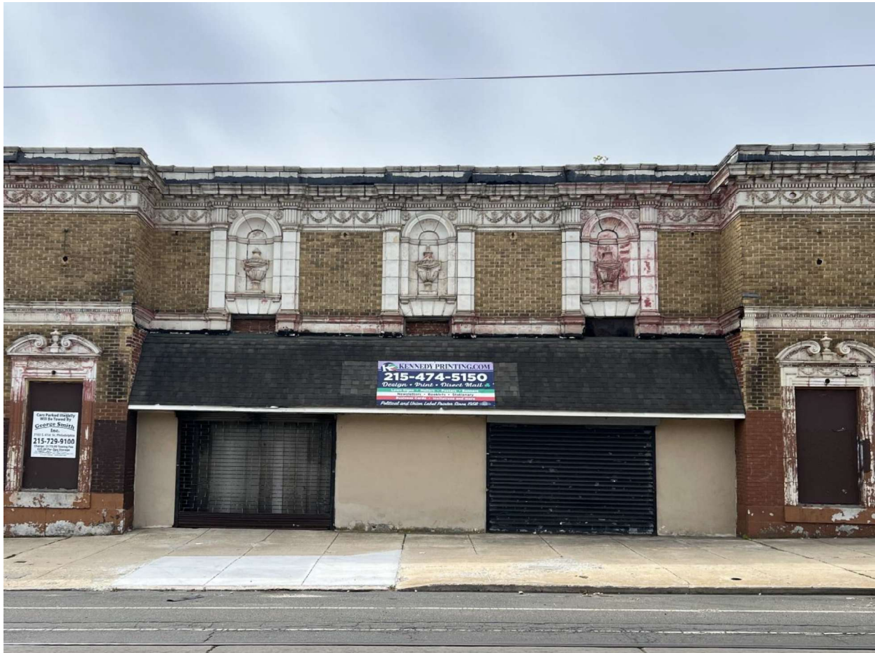
Figure 11: View of the facade's central volume.
