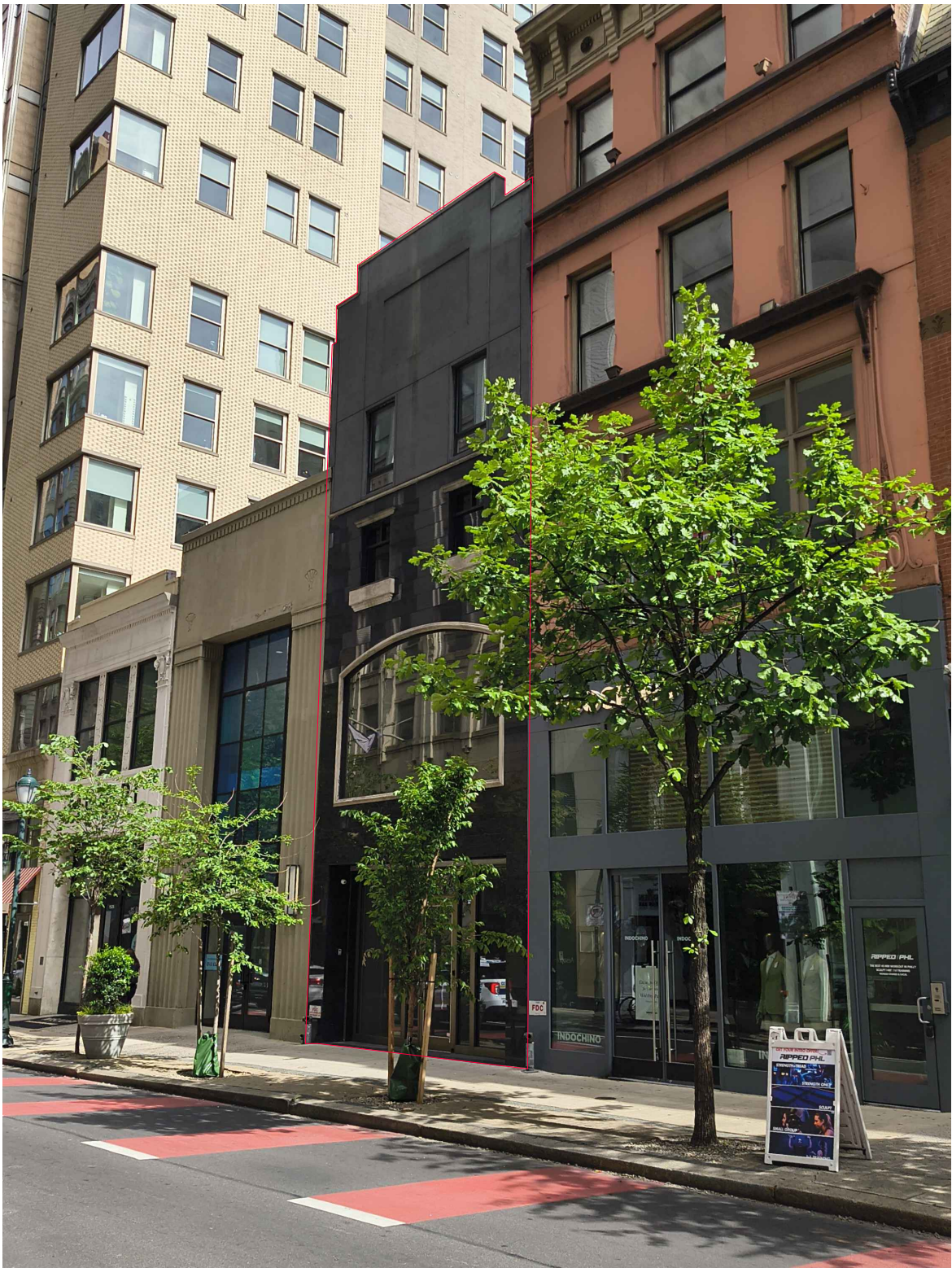
EXISTING FACADE - LATERAL VIEW
