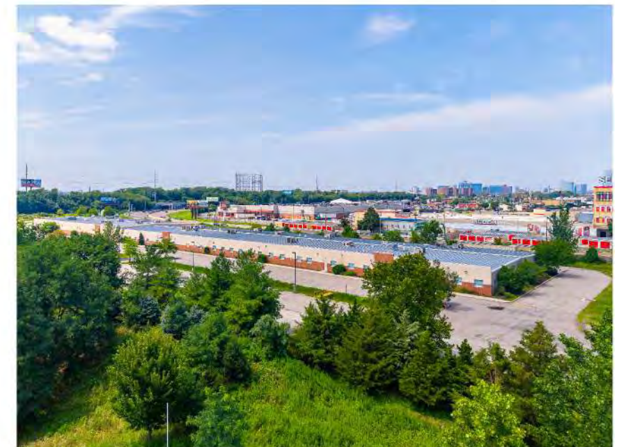
SITE PHOTO 2: LOOKING NW FROM SOUTH EAST CORNER OF SITE
