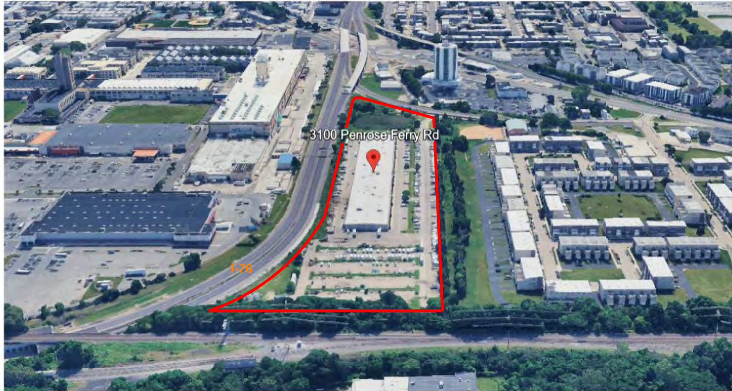
EXISTING AERIAL 3 - WEST
