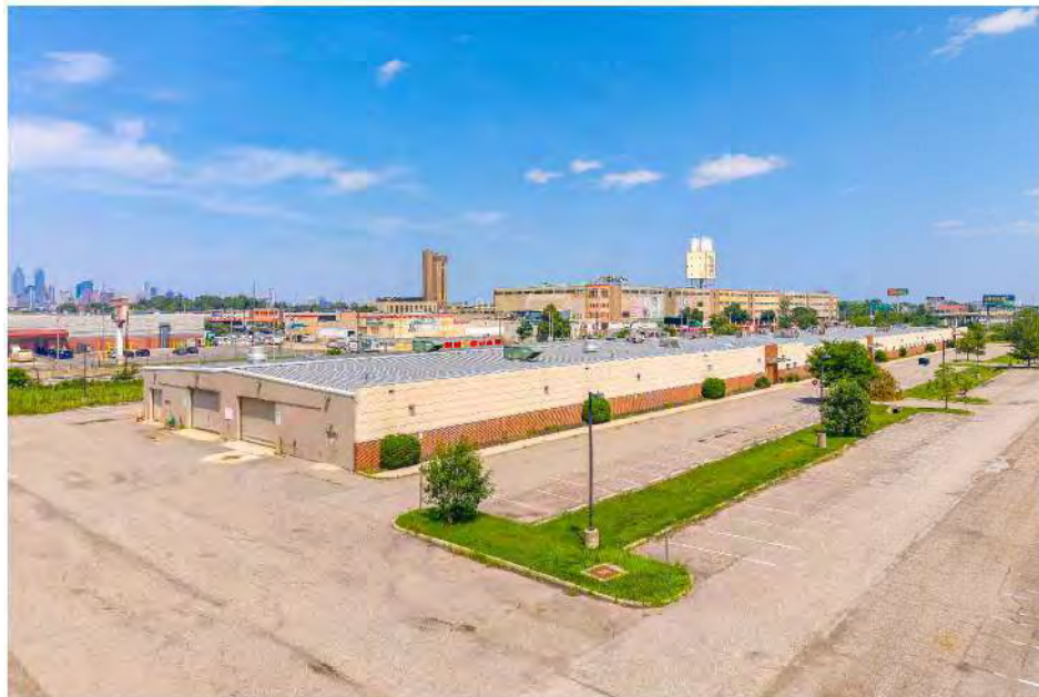
SITE PHOTO 3: LOOKING SOUTH - WEST SIDE OF EXISTING BUILDING
