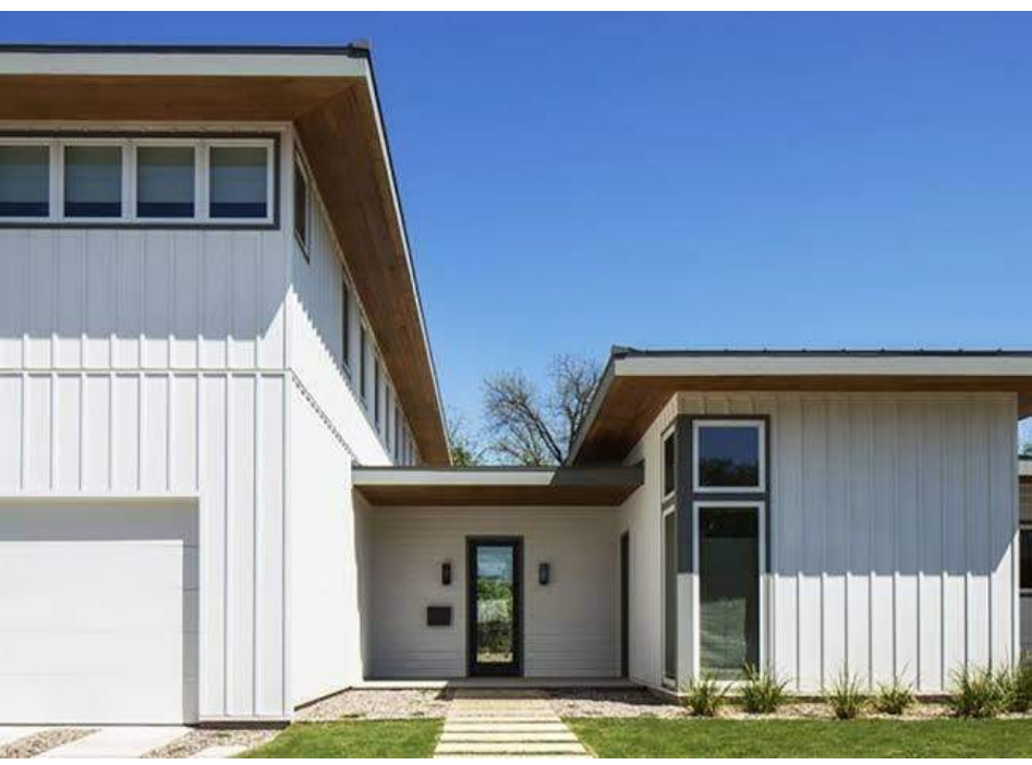
3-HARDI BOARD AND BATTEN
