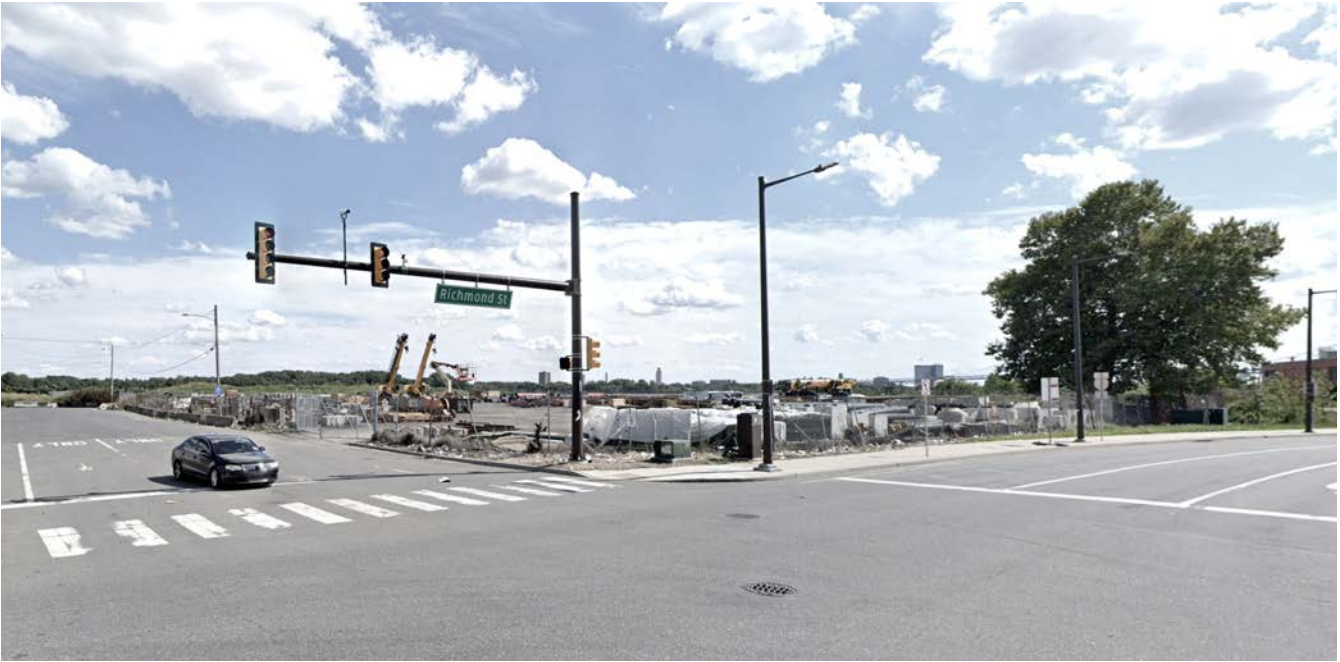
VIEW LOOKING S AT SCHIRRA + RICHMOND
