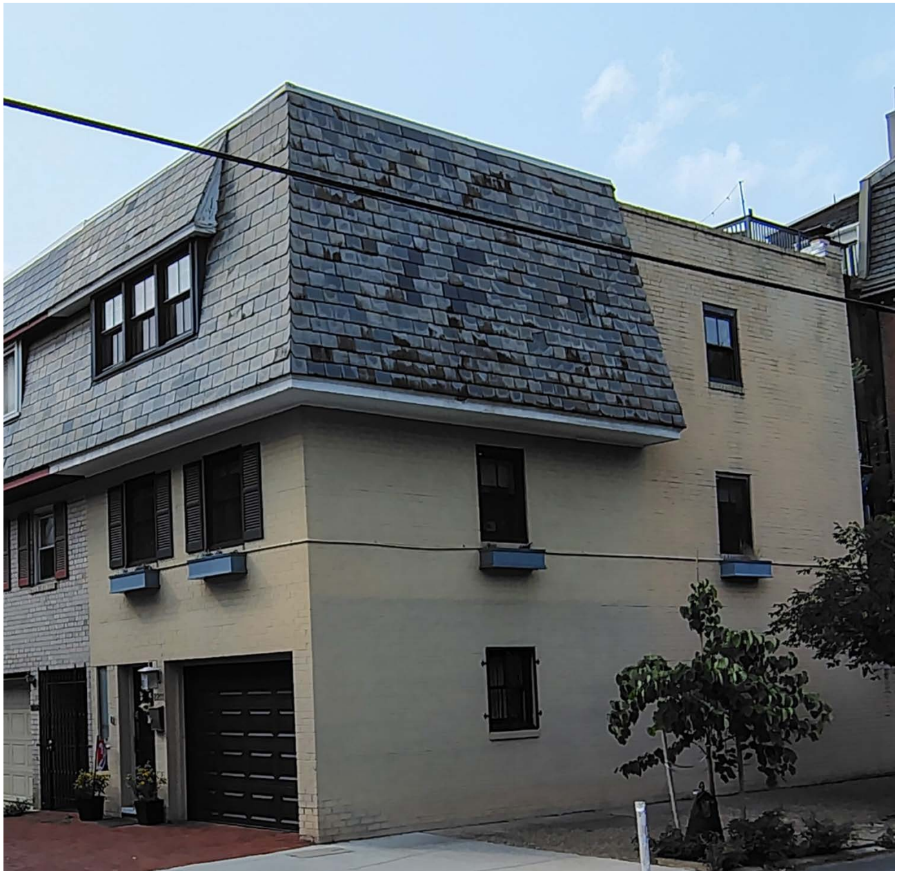
Figure 3: 2201 Panama St (Non-Contributing) Primary & East facades.
