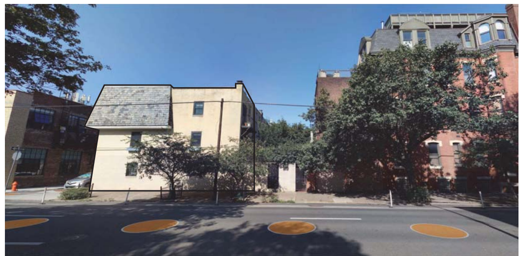
VIEW LOOKING WEST ON 22ND STREET
