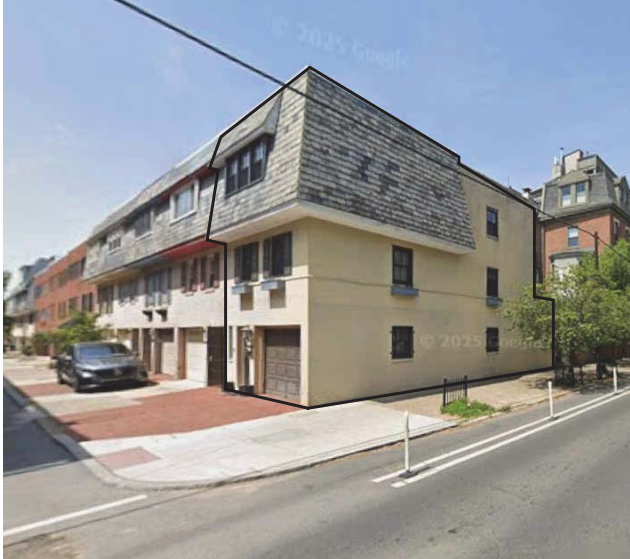
(EXIST) 2201 PANAMA ST. FRONT & SIDE FACADE
