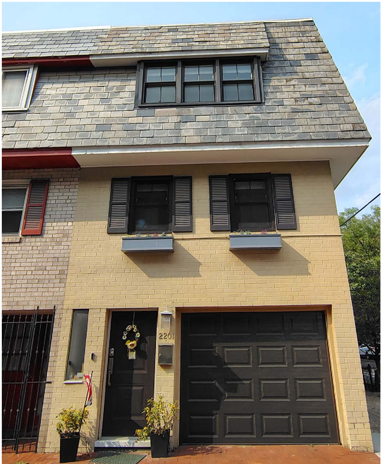
Figure 2: 2201 Panama St (Non-Contributing) Primary Façade.
