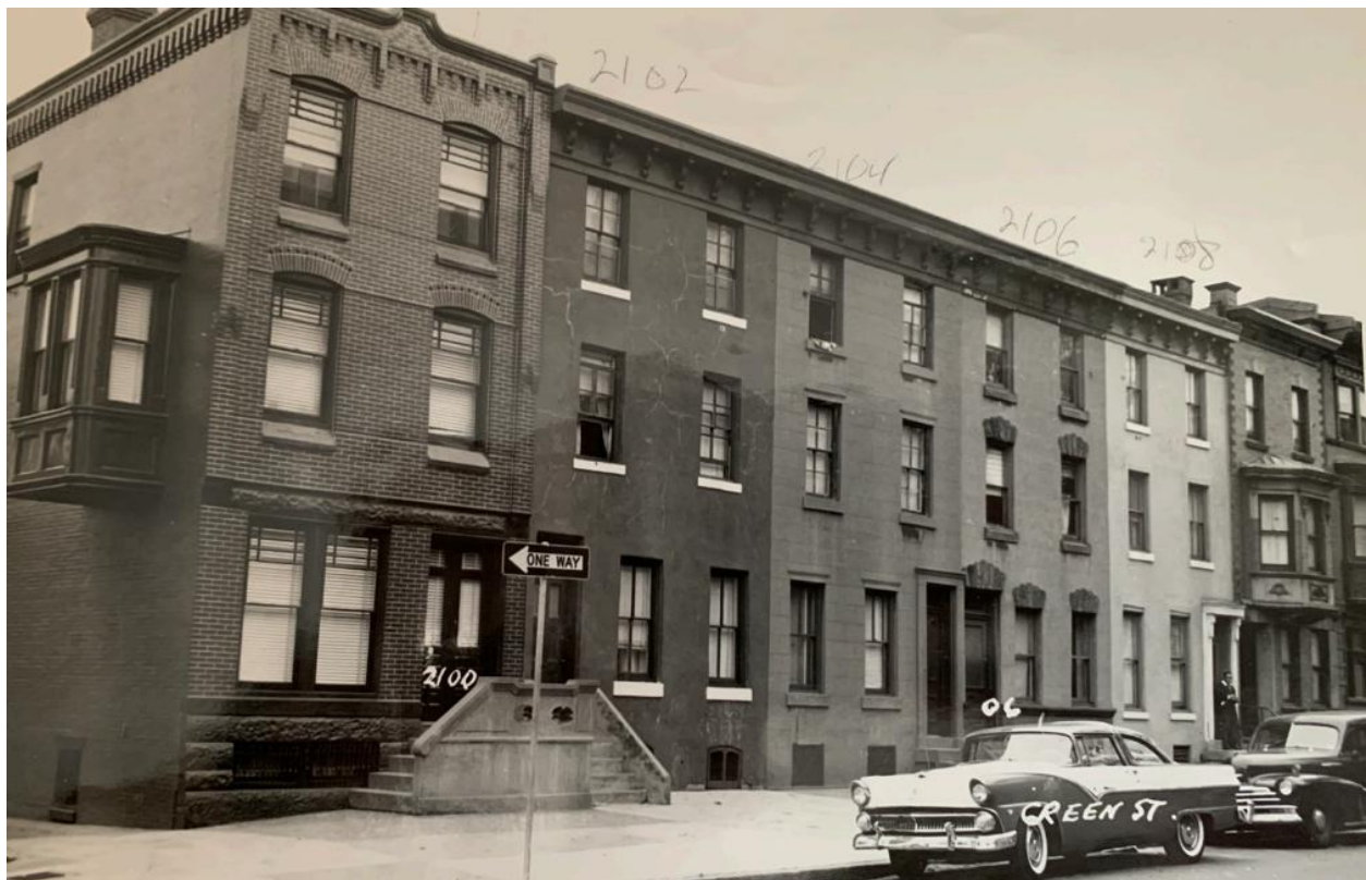
Figure 1. 2100-2110 Green Street, 1960. Source: PHC
