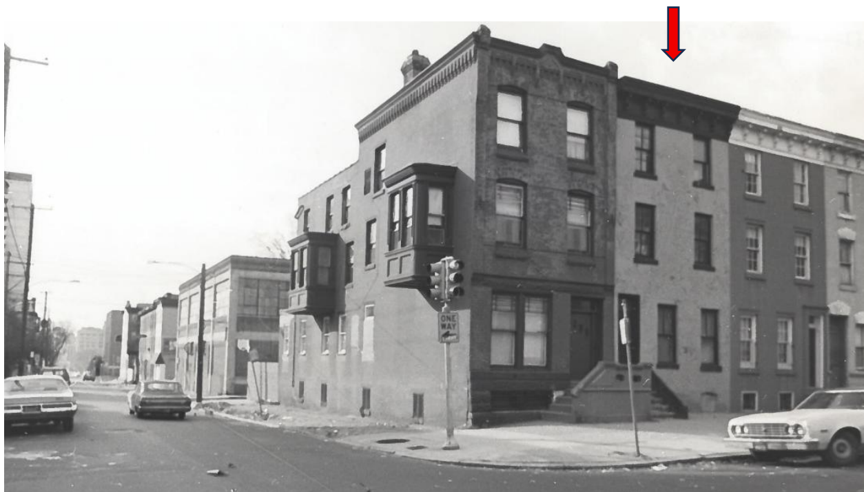
Figure 2. 2100-2104 Green Street, 1976. Source: PHC
