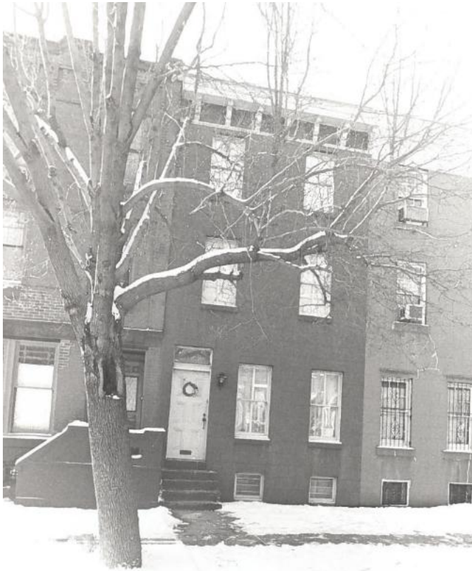
Figure 3. 2102 Green Street, 2001. Source: PHC
