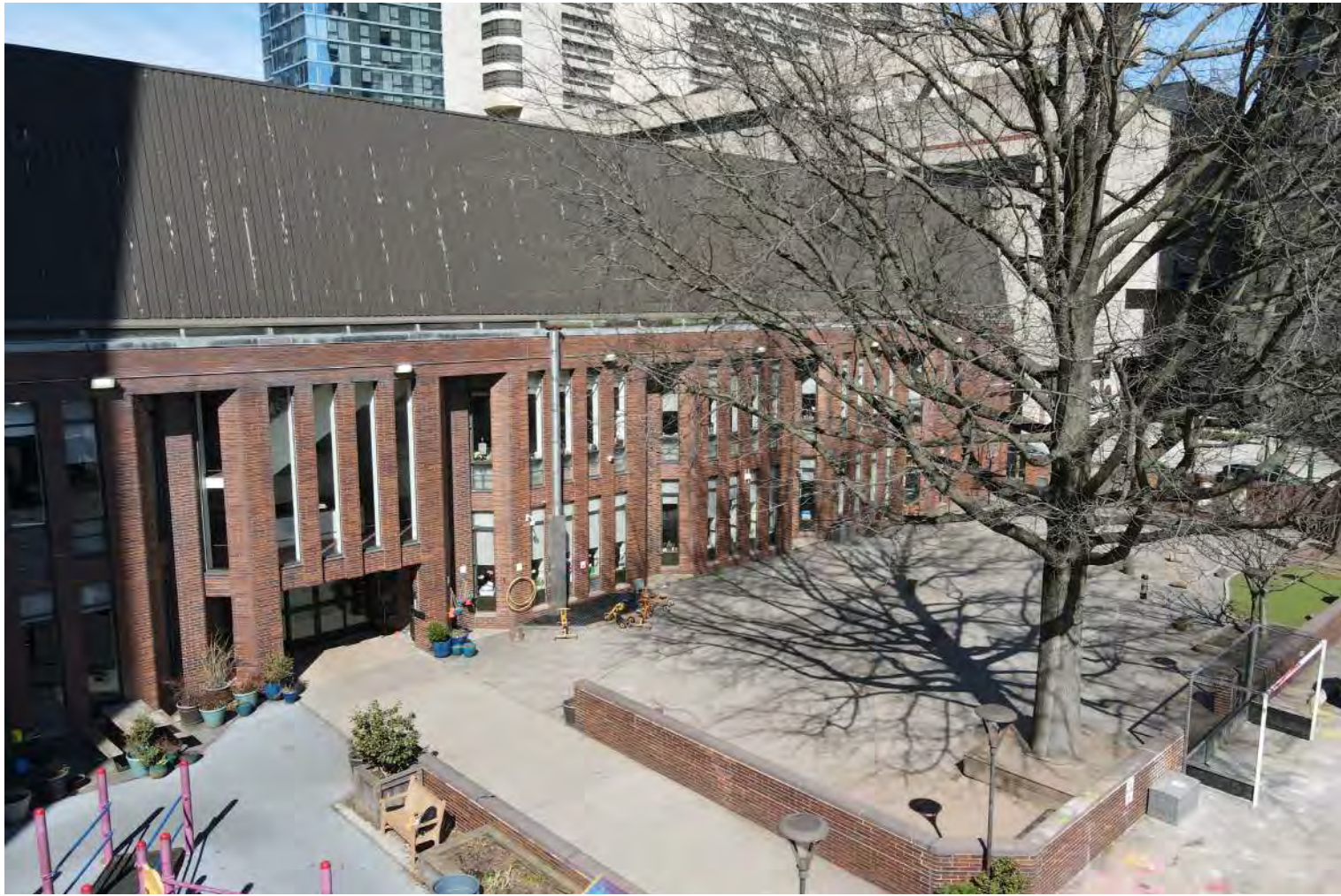
VIEW FROM BACKLOT LOOKING NORTHWEST (ROOF LEVEL)
