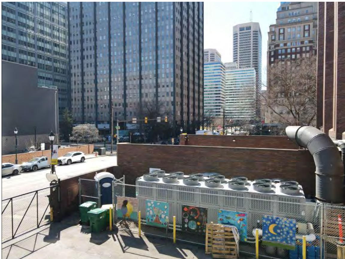
VIEW FROM SITE LOOKING SOUTHEAST DOWN 16TH STREET
