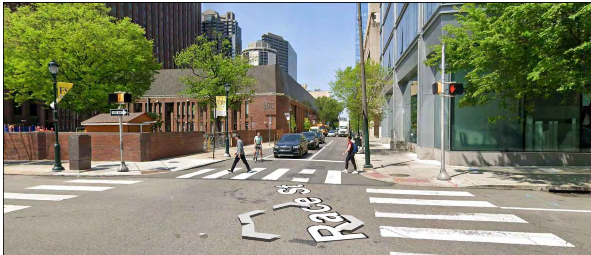
VIEW OF SITE, EXISTING VEHICLE GATE, AND ADJACENT BUILDINGS LOOKING WEST DOWN RACE STREET
