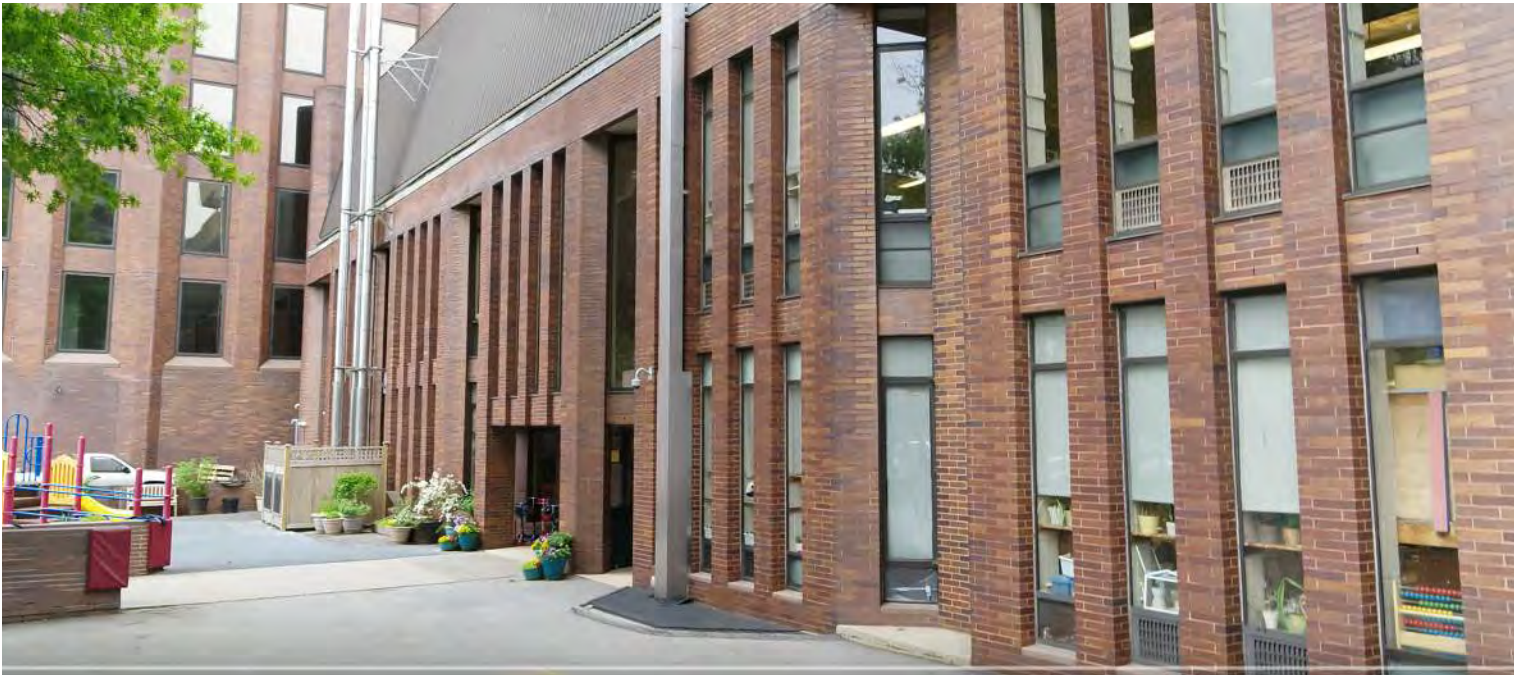
VIEW FROM BACKLOT LOOKING SOUTHWEST TOWARD SCHOOL
