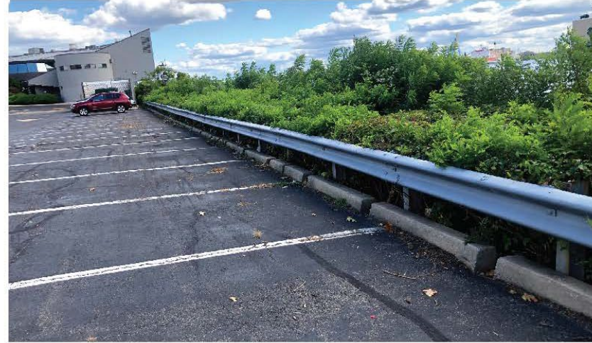
View looking East along parking lot
