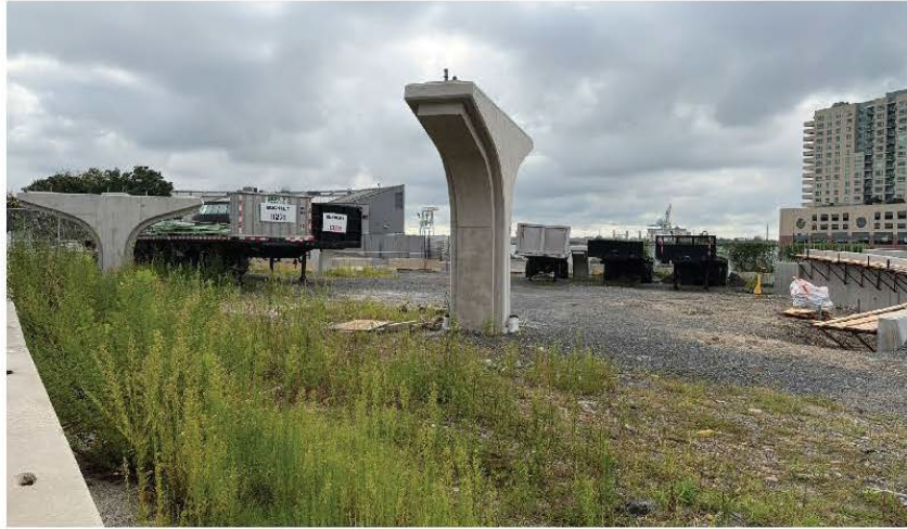
View of ramp support
