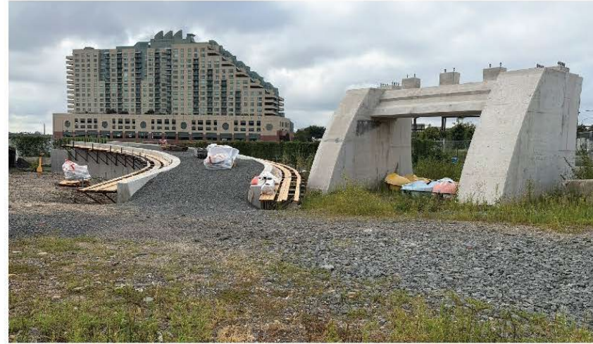
View of bridge support and ramp touchdown
