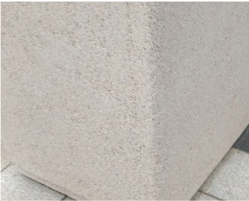
Concrete Base Precast
