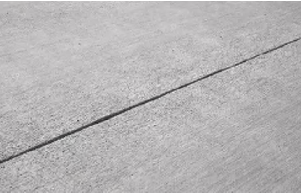
1 Concrete Paving Cast-in-place
