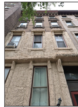
Photo B May, 2026 Detail of existing lower facade conditions
