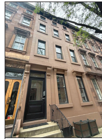
Photo D May, 2026 View of neighboring building 1514 Pine St. The existing neighboring building includes a stucco facade treatment with simulated masonry joints and ornament to match the original brownstone masonry.
