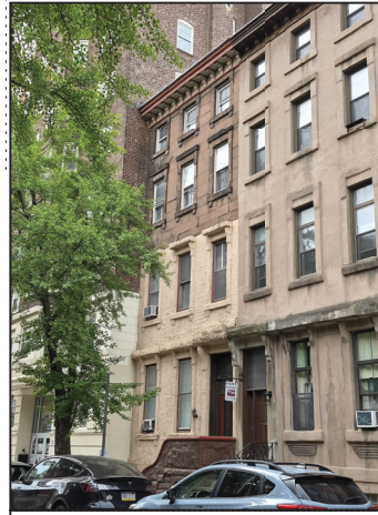
View of existing Pine St Facade
