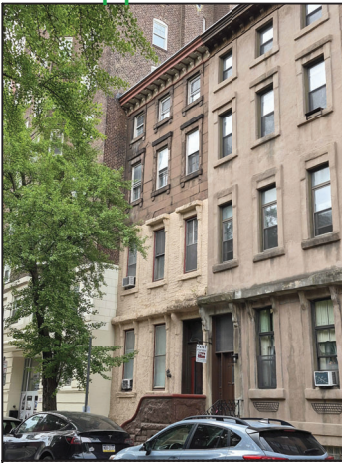
View of existing Pine St Facade
