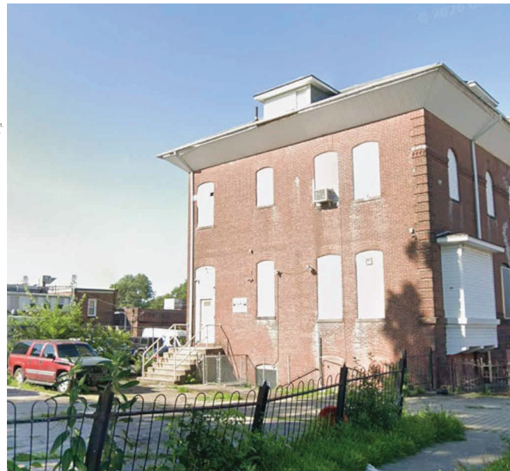
Parking lot elevation. Primary area of work.
