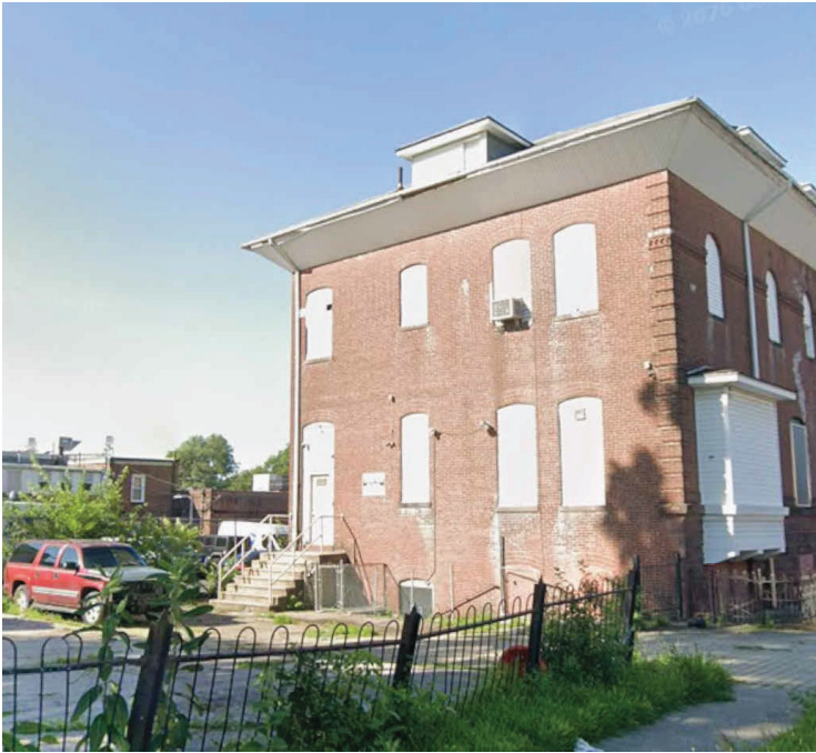
Parking lot elevation. Primary area of work.
