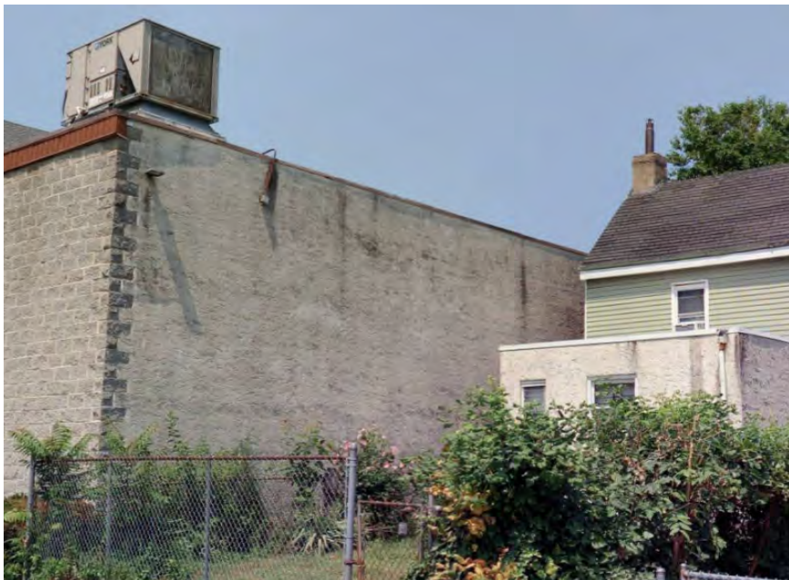
Image 14. Southeast facade as viewed from Meadow Street. Image from July 2025, cyclomedia.gov.
