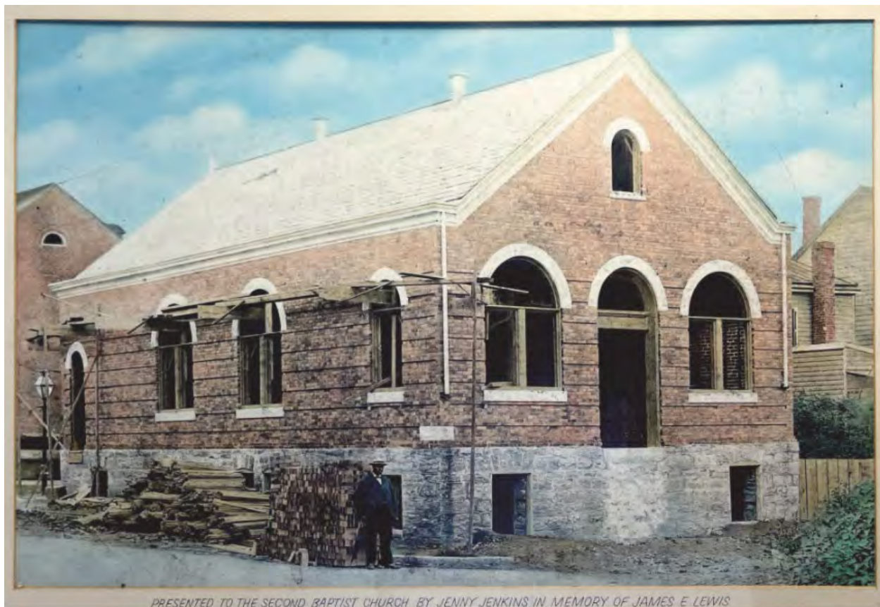
Image 17. Likely colorized print of photograph of 1905-06 building, under construction. c. 1905-06. Courtesy of Second Baptist Church of Frankford.
