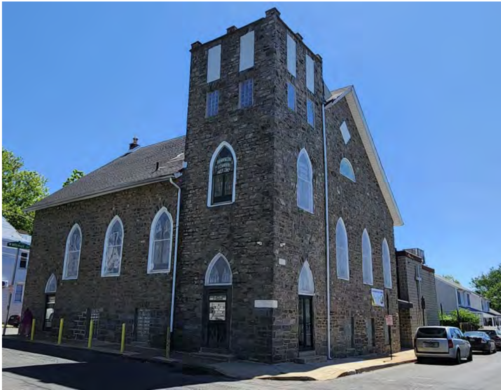
Image 1. View of Second Baptist Church of Frankford from intersection of Mulberry and Meadow Streets. Photo by PHC staff, 2026.
