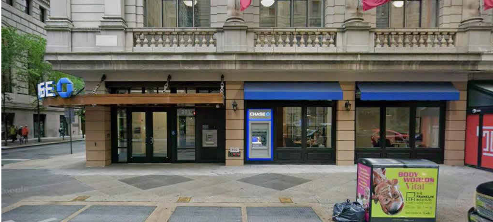
VIEW LOOKING AT NORTH END OF BUILDING
