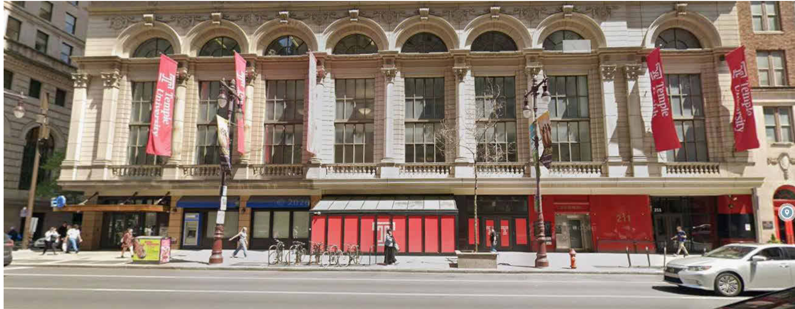
OVERALL BUILDING STREET VIEW
