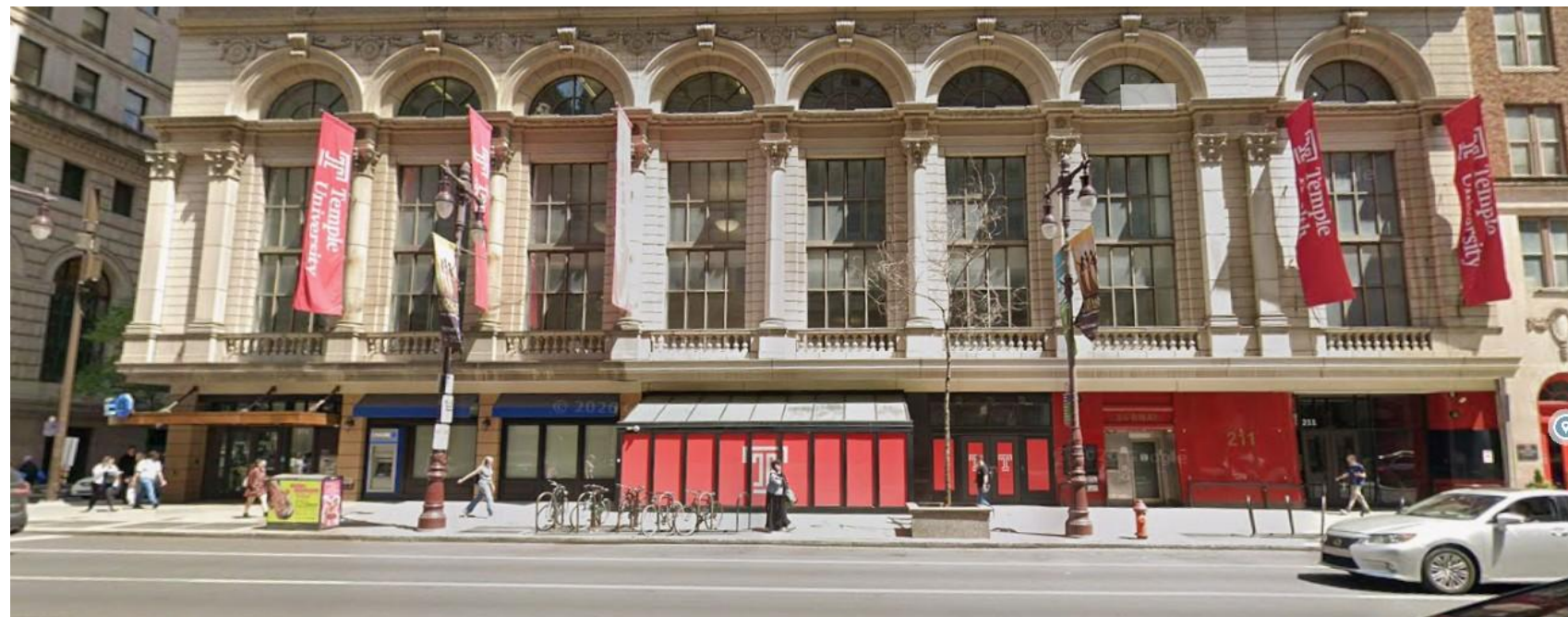
VIEW FROM ACROSS THE STREET
