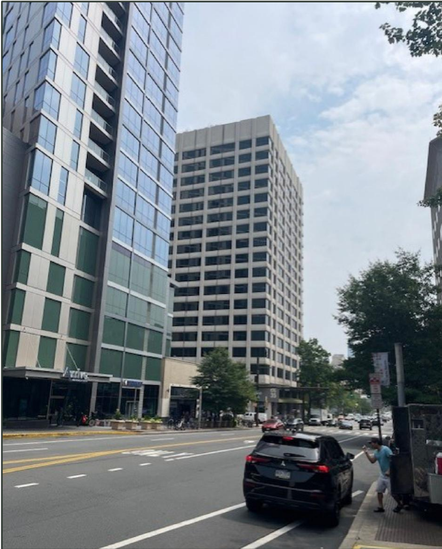
West Building Face – Existing Condition View from Market Street facing east
