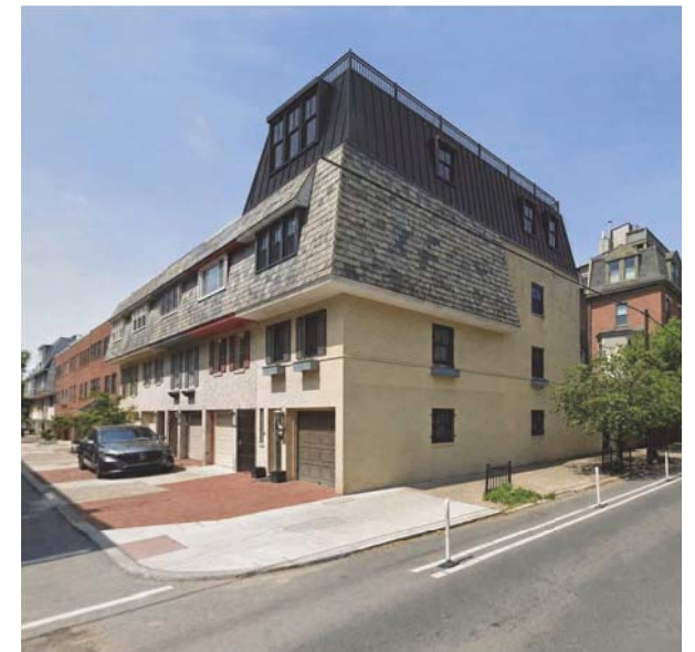
VIEW LOOKING WEST ON 22nd STREET
