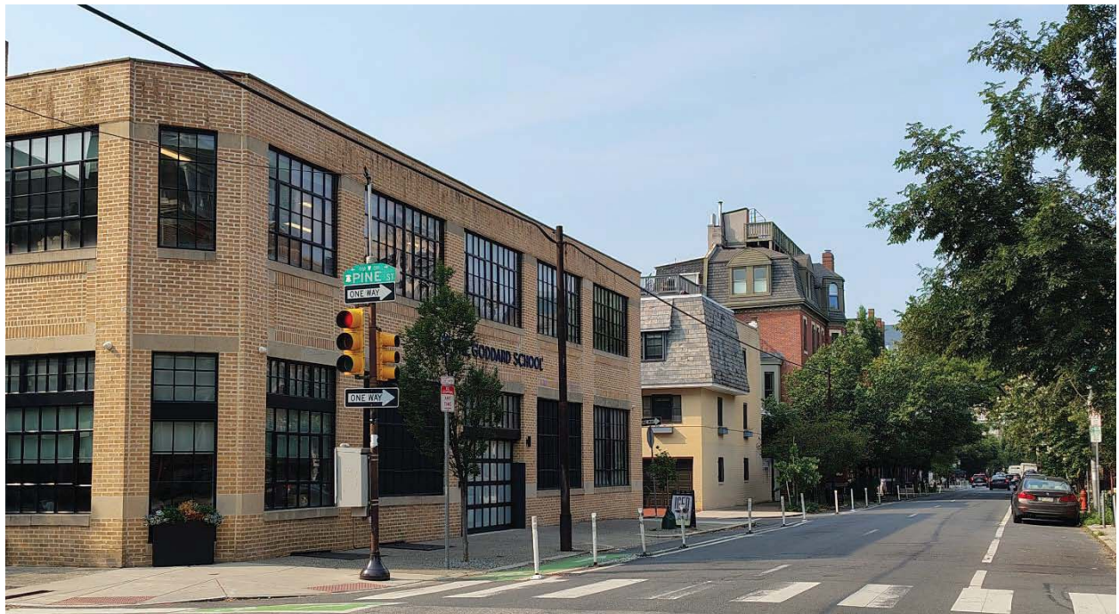
Figure 5: Looking North on 22 nd St. 2201 Panama St (Non-Contributing) on left, center.
