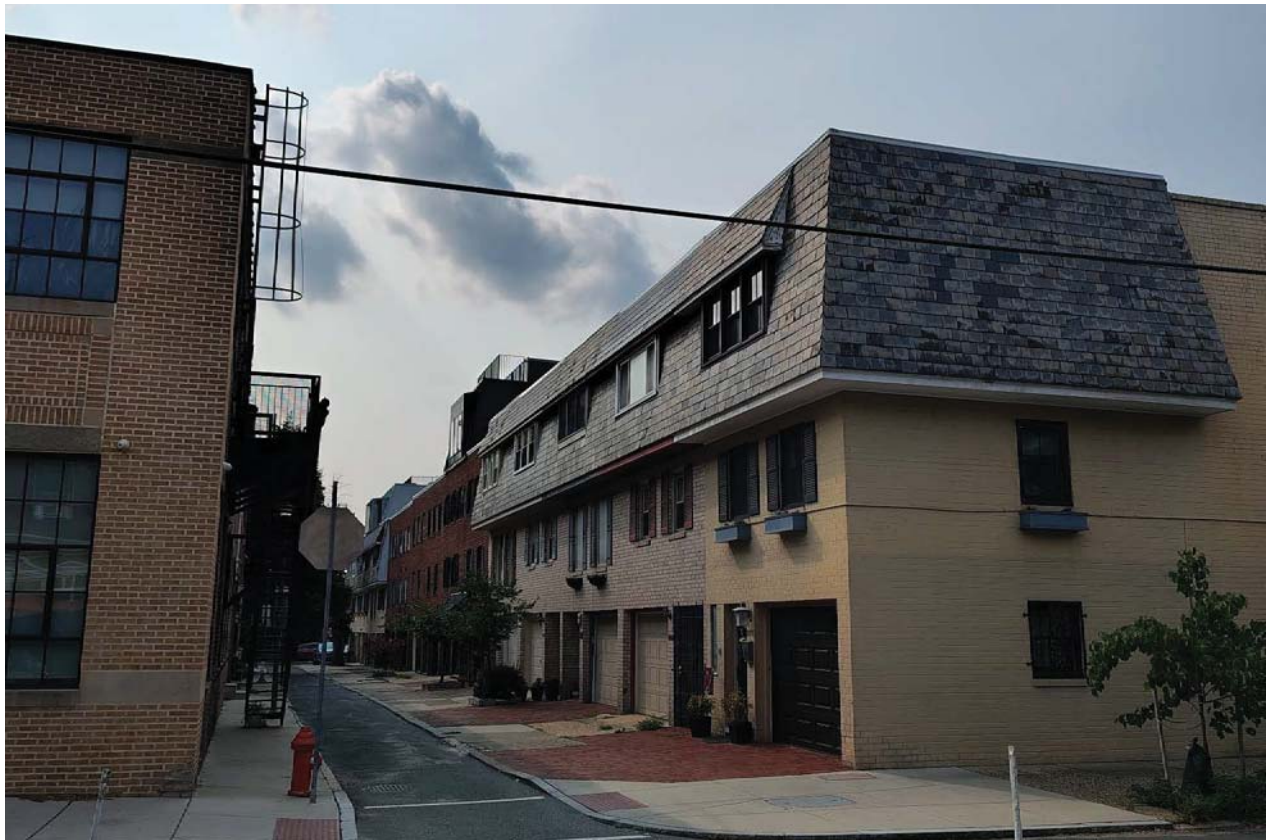
Figure 4: Looking west on Panama St, 2201 Panama St (Non-Contributing) on right.
