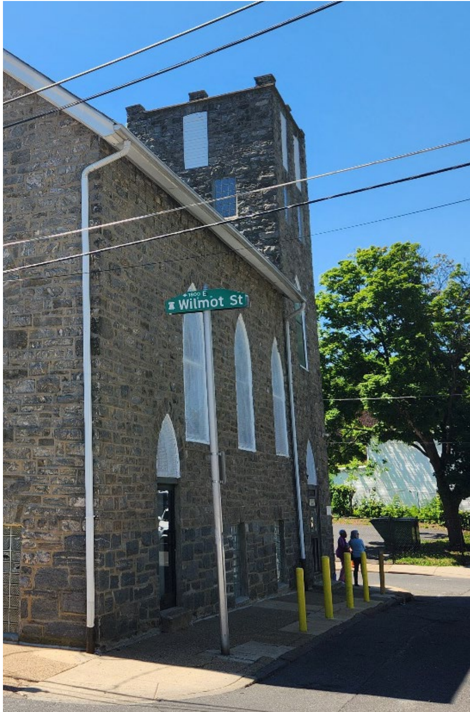
Image 6. Showing northeast side of tower, as viewed from intersection of Mulberry and Wilmot Streets. Photograph by nominator, June 4, 2026.
