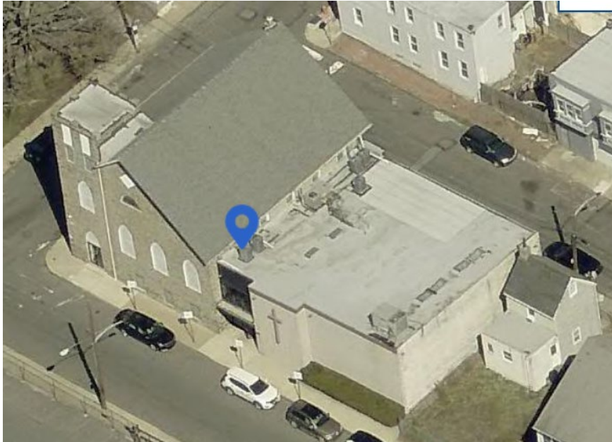
Image 13. Aerial view of southeast elevations, showing extent of encapsulation of the historic wall in the 1991 addition. Image from March 2025, pictometry.phila.gov.
