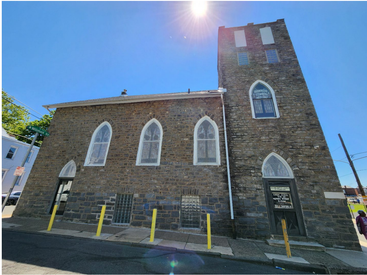
Image 5. Northwest facade (Mulberry Street). Taken by nominator, June 4, 2026.
