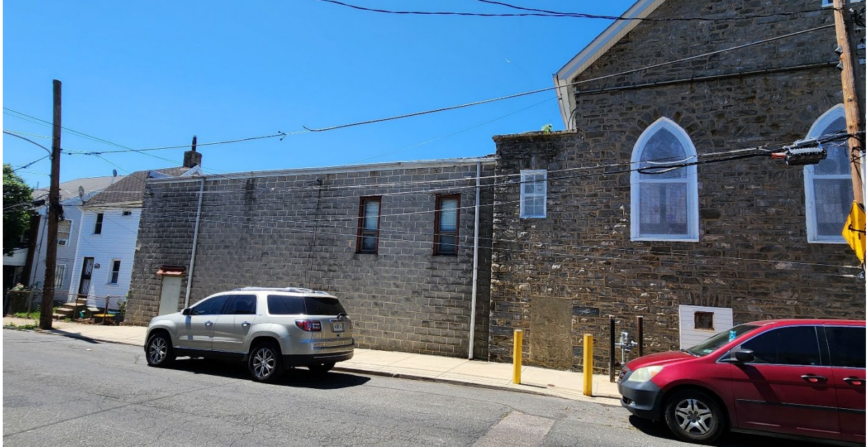
Image 12. Northeast facade of non-historic addition (Wilmot Street). Photograph by nominator, June 4, 2026.
