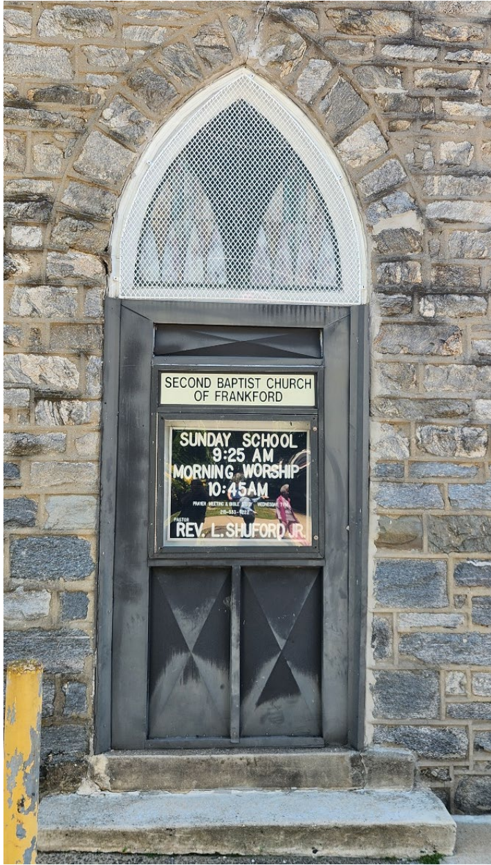
Image 8. Infilled doorway, northwest facade at base of tower. Photograph by nominator, June 4, 2026.
