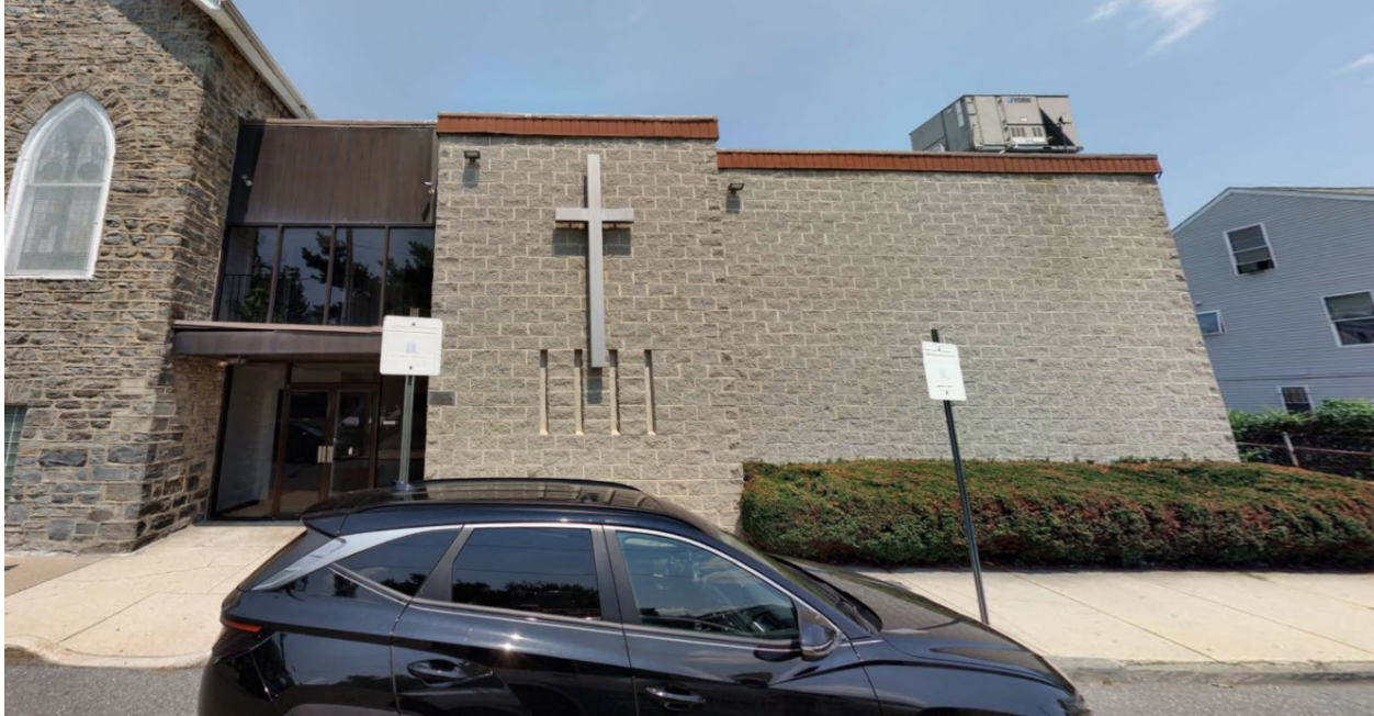
Image 4. Non-historic addition, southwest façade (Meadow Street), August 2025 image, cyclomedia.gov.
