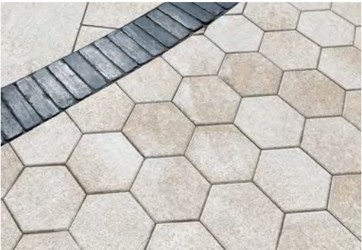
PRECAST CONCRETE UNIT PAVING
