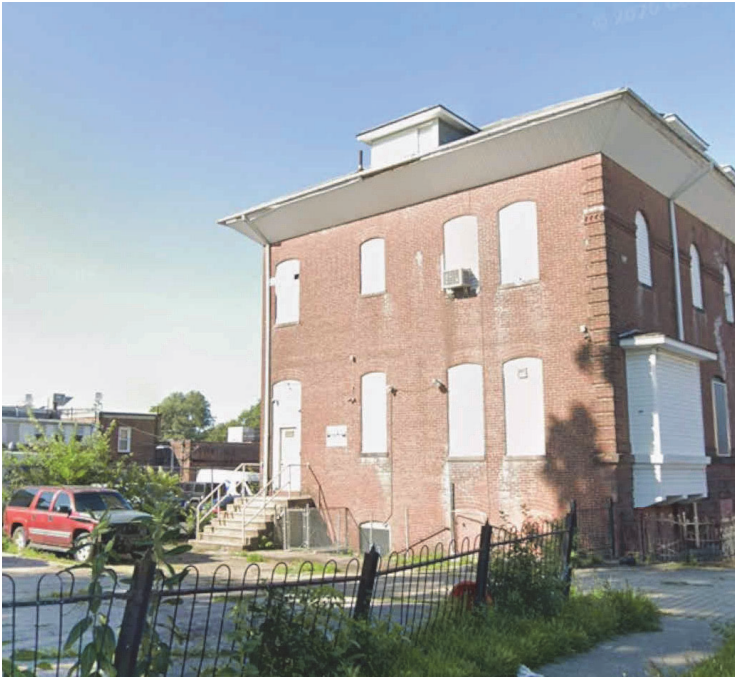
Parking lot elevation. Primary area of work.
