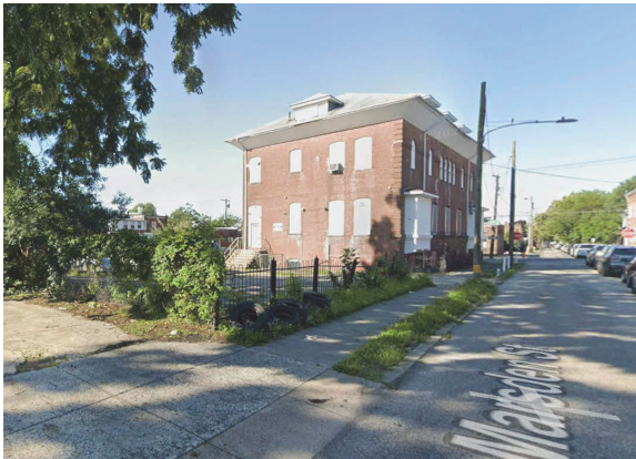
NE Corner. Parking lot shown in foreground.
