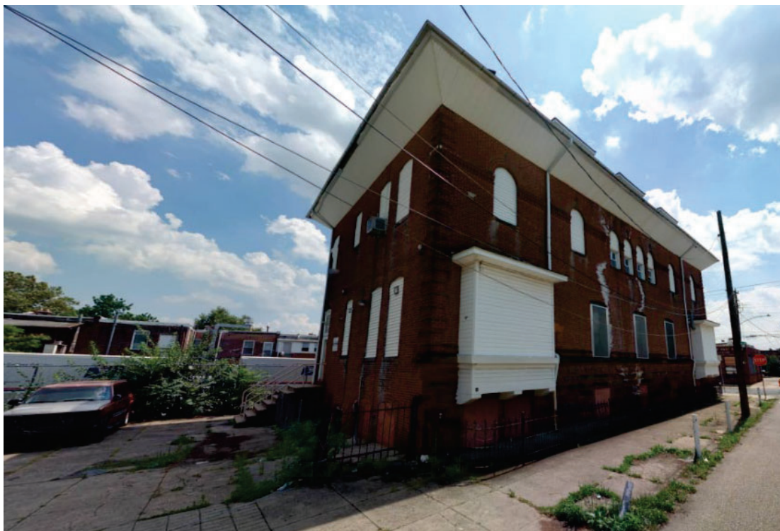
Figure 5: View from Marsden Street (facing south) of rear and side elevations.
