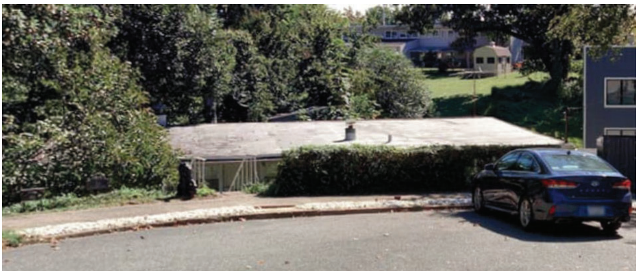
Image 2: Front façade as viewed from the cul-de-sac at the end of Longford Street.
