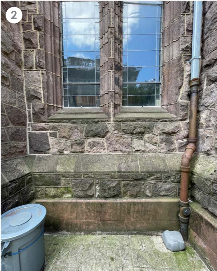
Base of exterior walls at location of future opening
