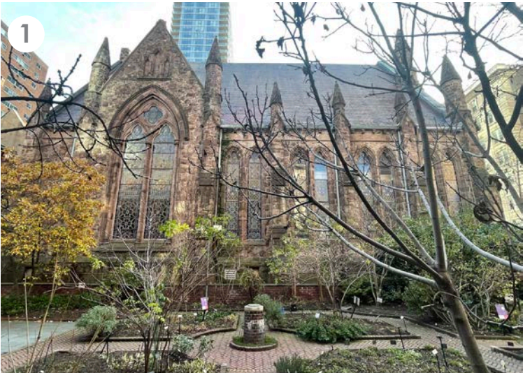
North Elevation, facing Courtyard
