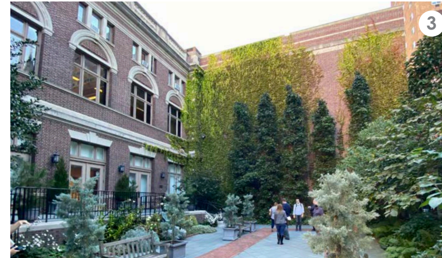
West Elevation, along 22nd Street
