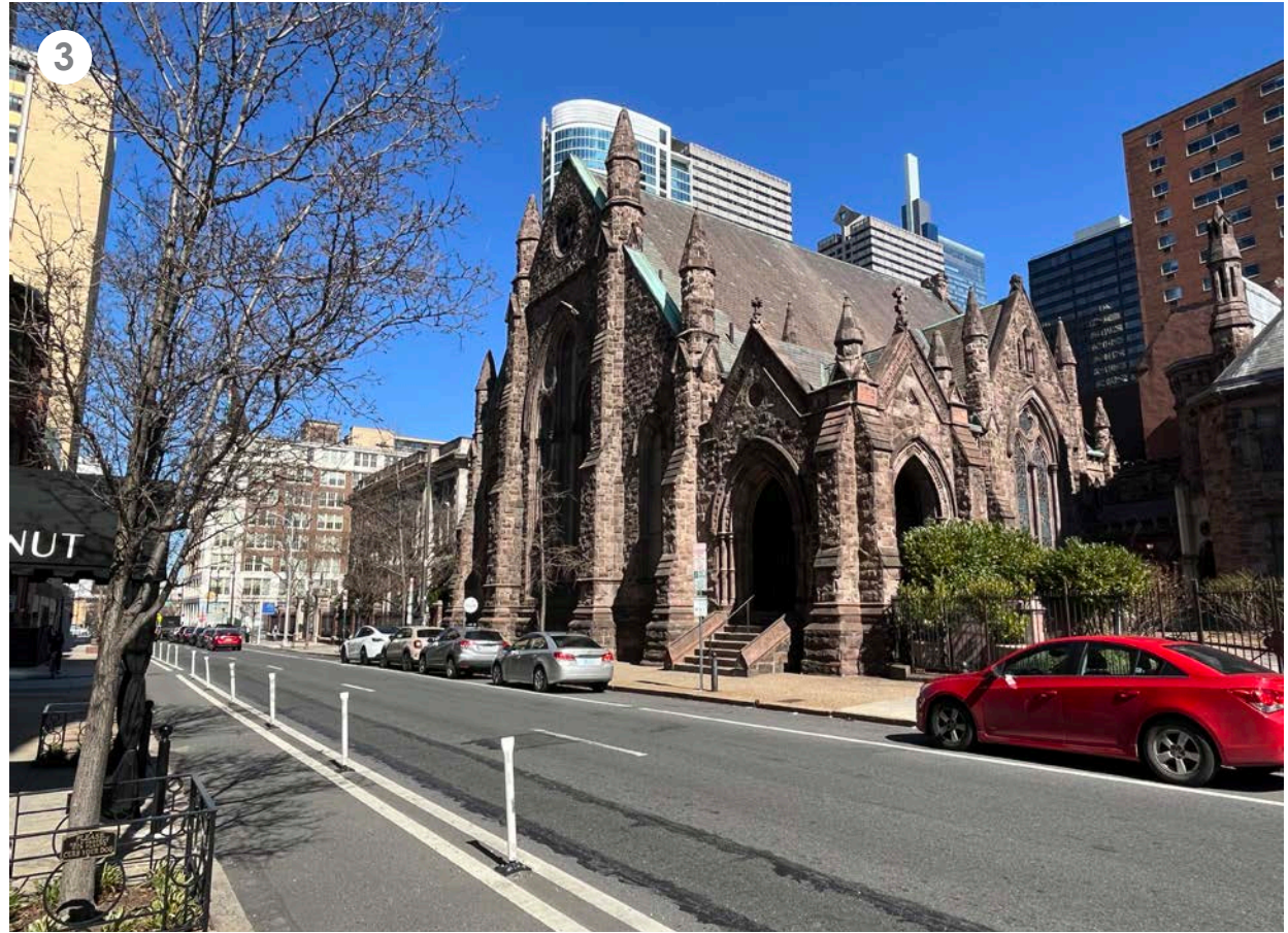
West Elevation, along 22nd Street
