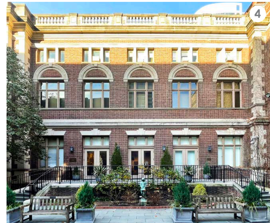
South Elevation, outside Thomson
