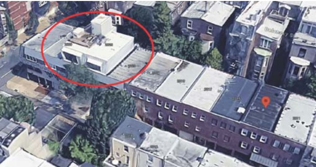
2225-2227 PANAMA ST MANSARD ADDITION
