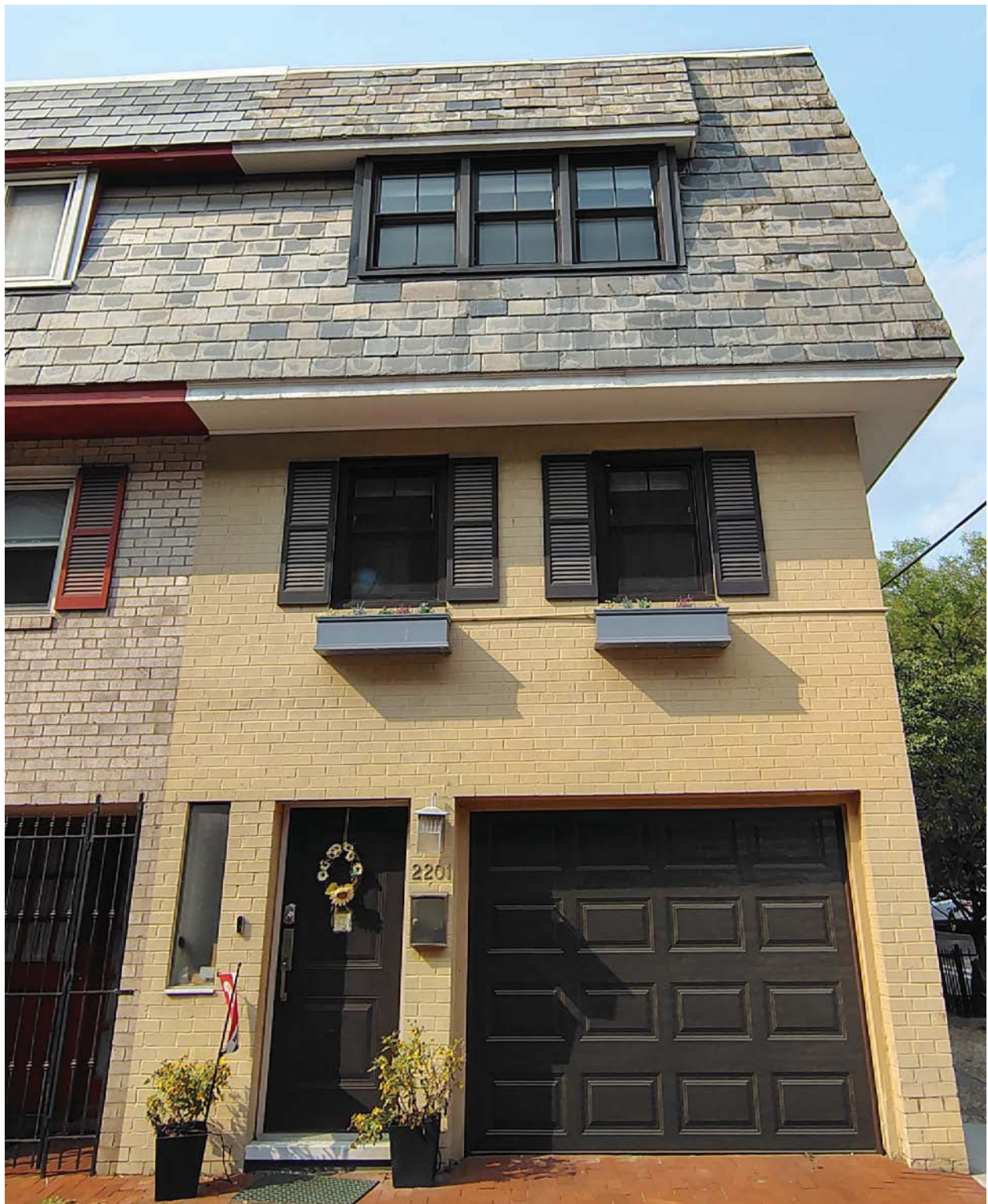
Figure 2: 2201 Panama St (Non-Contributing) Primary Façade.
