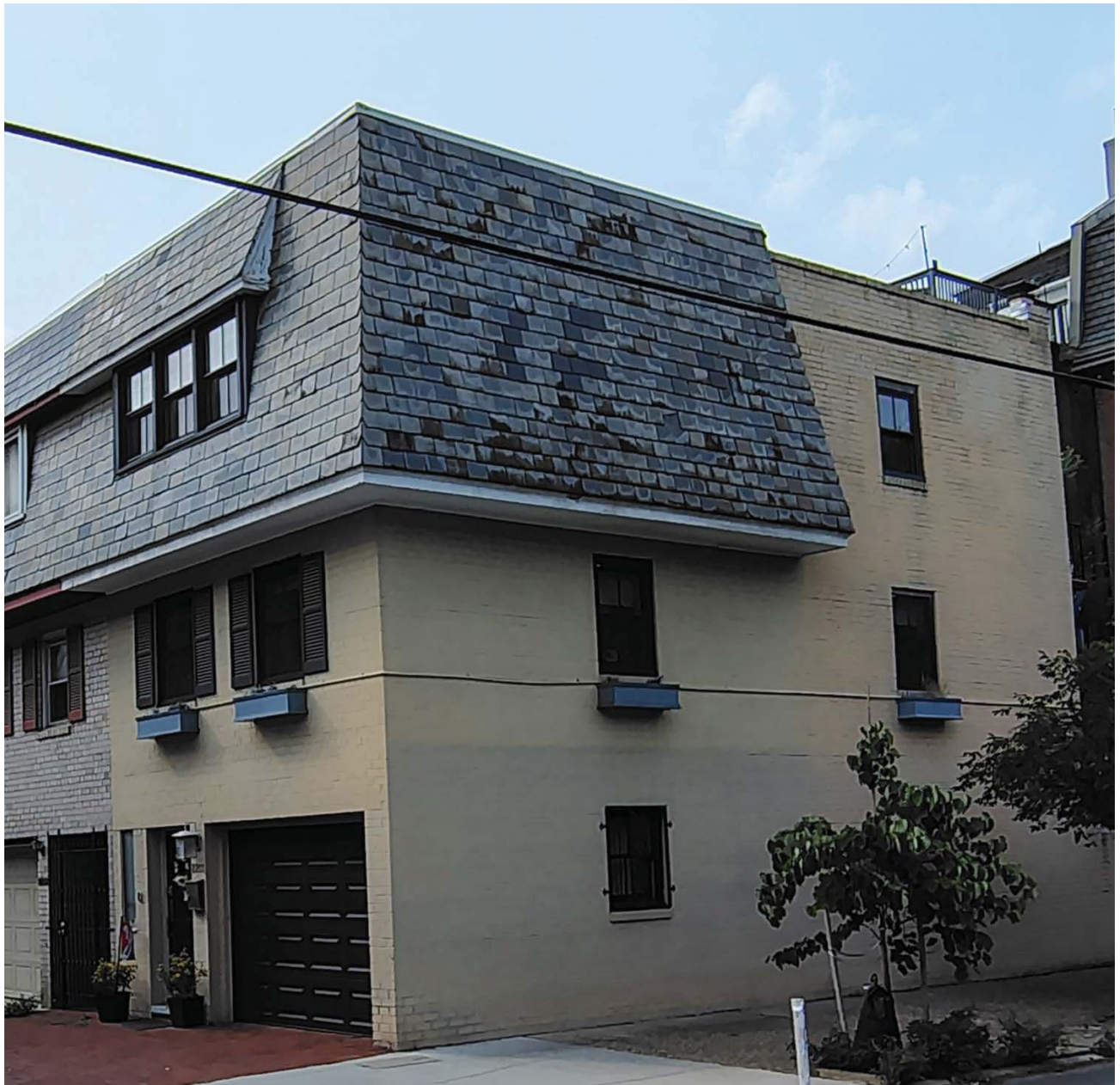
Figure 3: 2201 Panama St (Non-Contributing) Primary & East facades.
