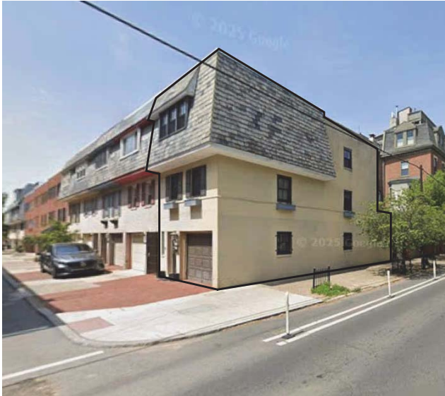
(EXIST) 2201 PANAMA ST. FRONT & SIDE FACADE
