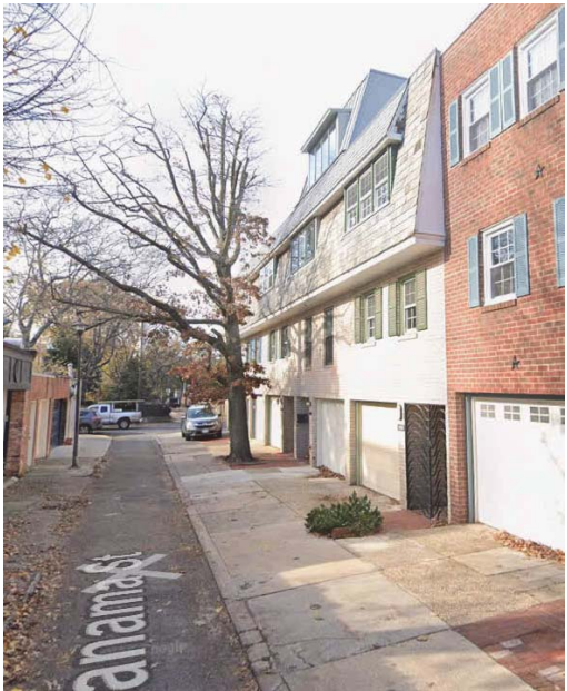
2225 PANAMA ST MANSARD ADDITION
