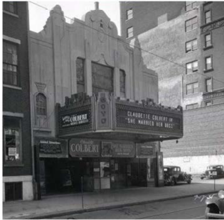
Historical Facade Marquee Condition
