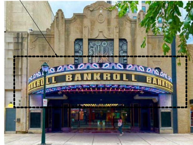
Recent Facade Marquee Condition
