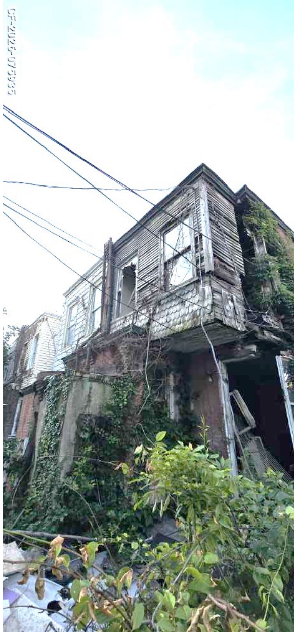
Figure 3. Department of Licenses and Inspections photograph of the rear of rear ell at 4275 Viola Street from CF-2026-075935.
