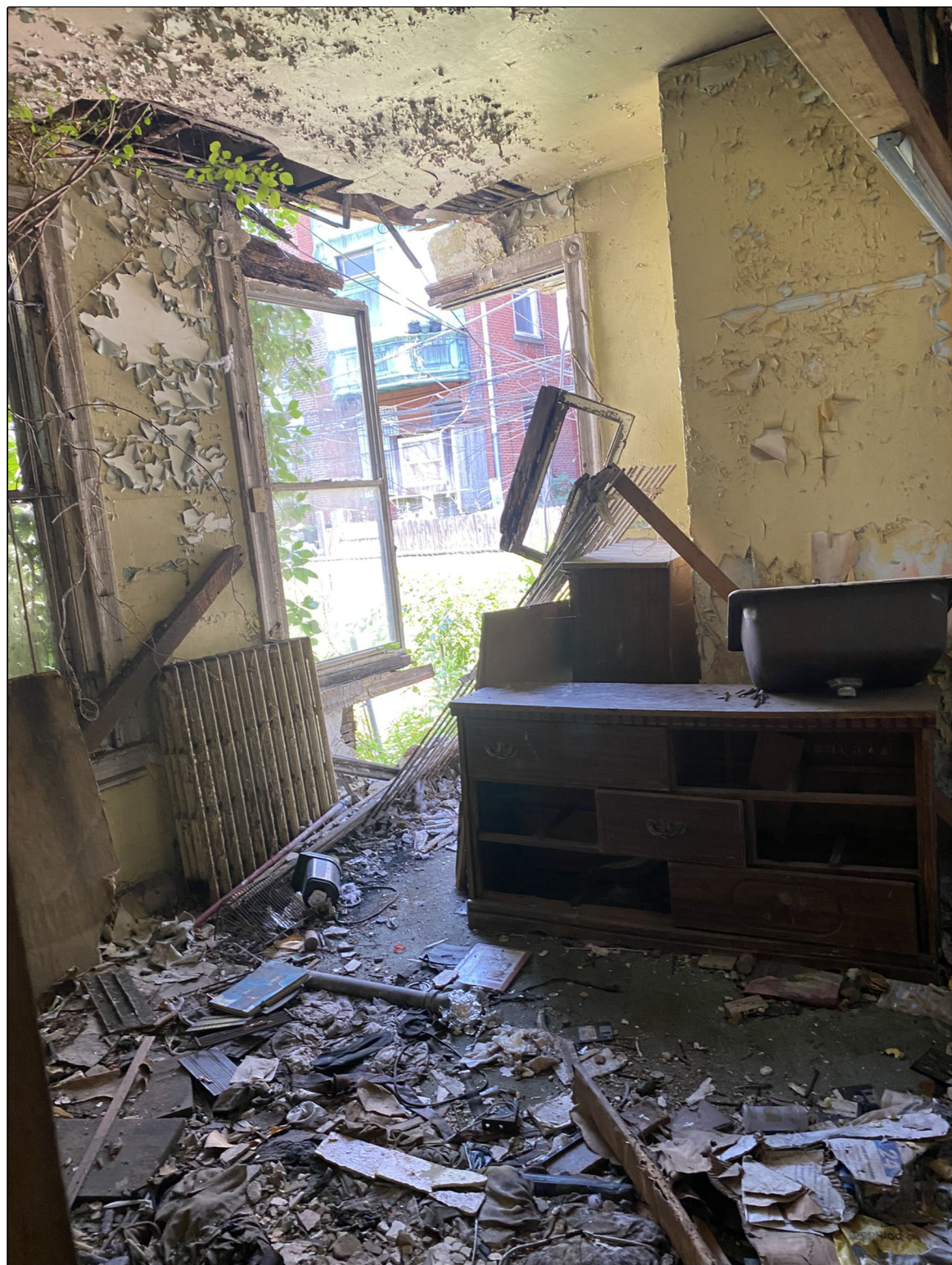
2 Interior Conditions (4275 Viola St) N.T.S.
