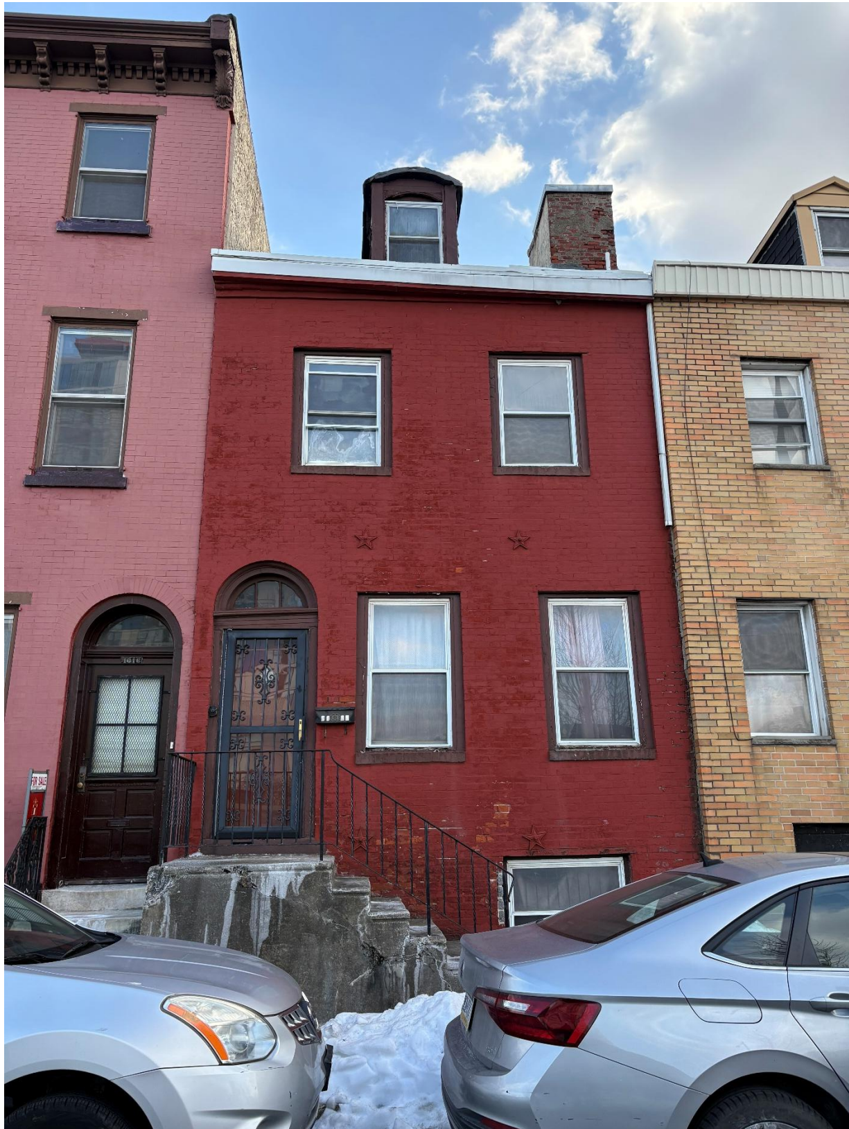
Image 6: Front façade of 1018 Winter Street, 2026. Historical Commission, 2026.
