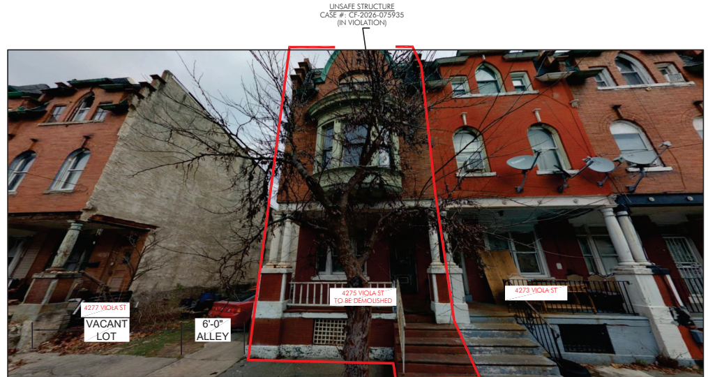
SUBJECT OF DEMOLITION REFERENCE PICTURE OF FRONT WITH TREE WITHOUT LEAVES TAKEN FROM CITY OF PHILADELPHIA ATLAS- DATED DEC. 19, 2022
