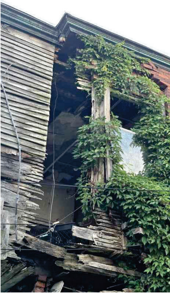
Figure 4. Department of Licenses and Inspections photograph of the rear of rear ell at 4275 Viola Street from CF-2026-075935.
