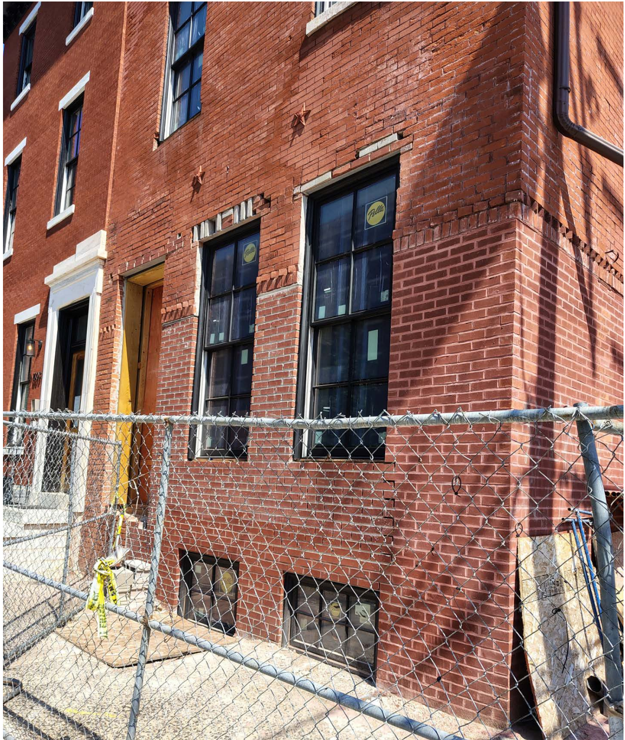
Figure 2: Current first floor restoration under construction.
