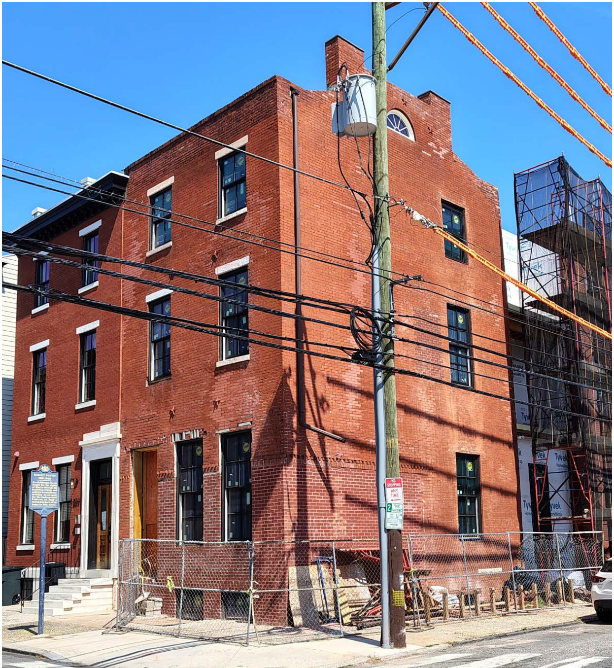
Figure 1: Current South (primary) façade and east façade under rehabilitation.
