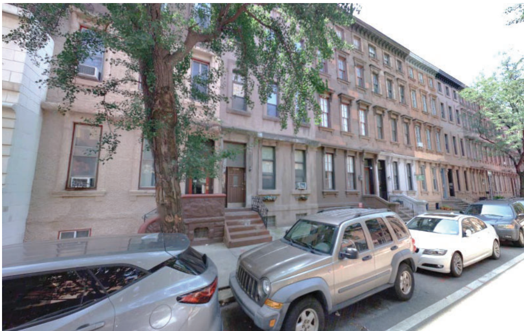
Figure 4: Subject property, at left, is at the end of the row of 18 brownstone rowhouses.
