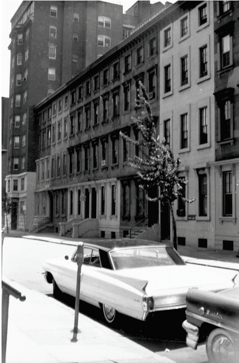
Figure 9: 1964 photograph showing the row before it was listed on the Philadelphia Register of Historic Places. Several houses had already been significantly altered.
