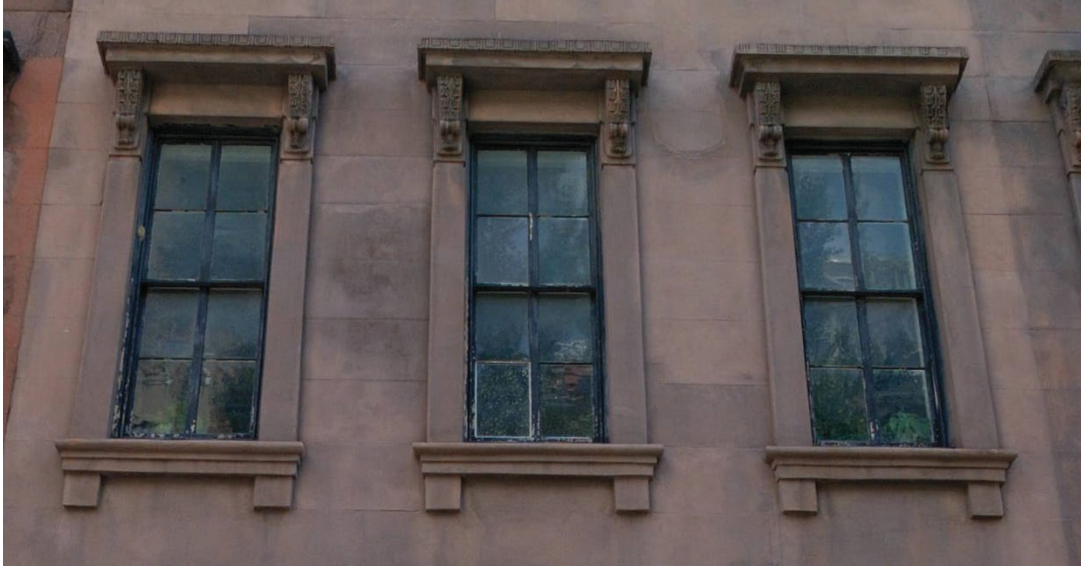
Figure 7: Surviving second-floor detail at 1522 Pine Street.
