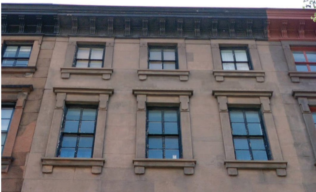
Figure 8: Third- and fourth-floor window trim in good condition at 1522 Pine Street.
