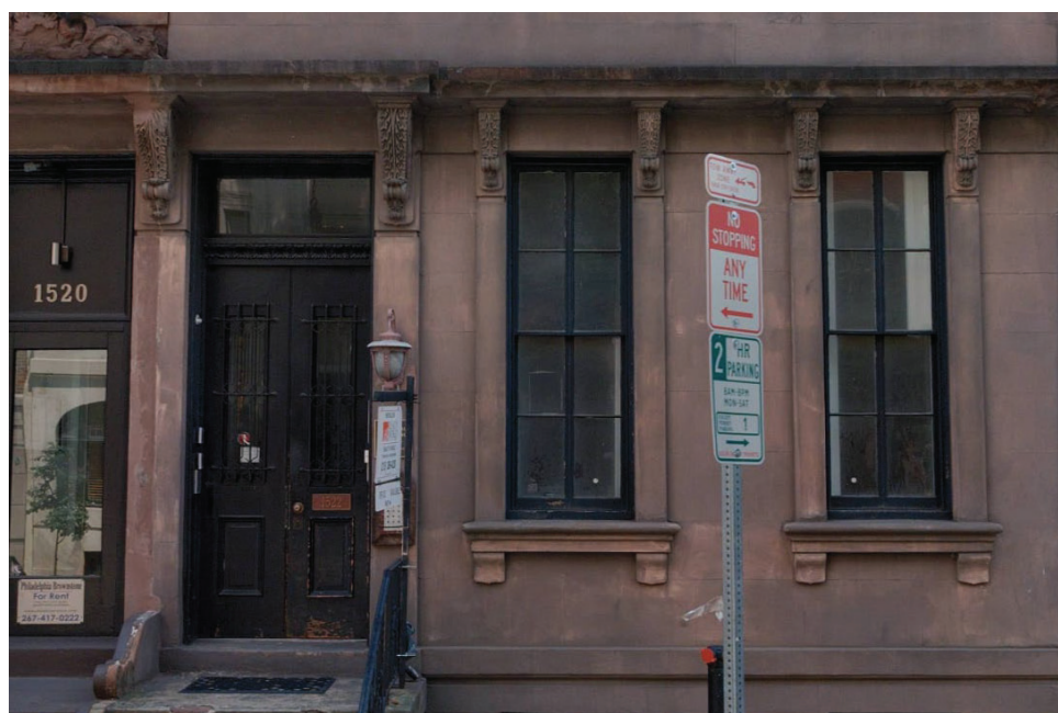
Figure 6: Surviving first-floor details at 1522 Pine Street.
