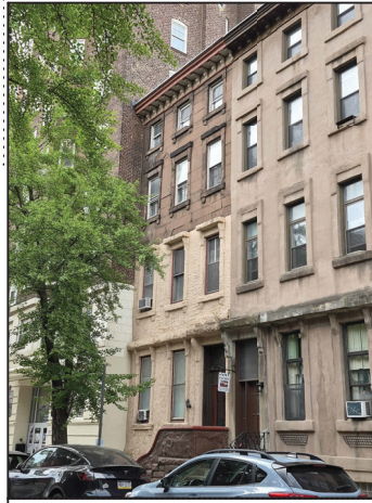
View of existing Pine St Facade
