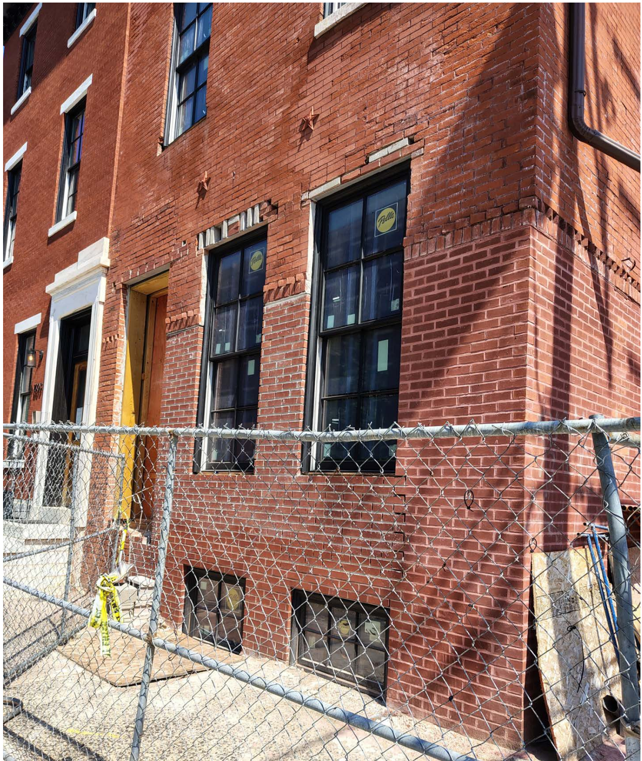
Figure 2: Current first floor restoration under construction.
