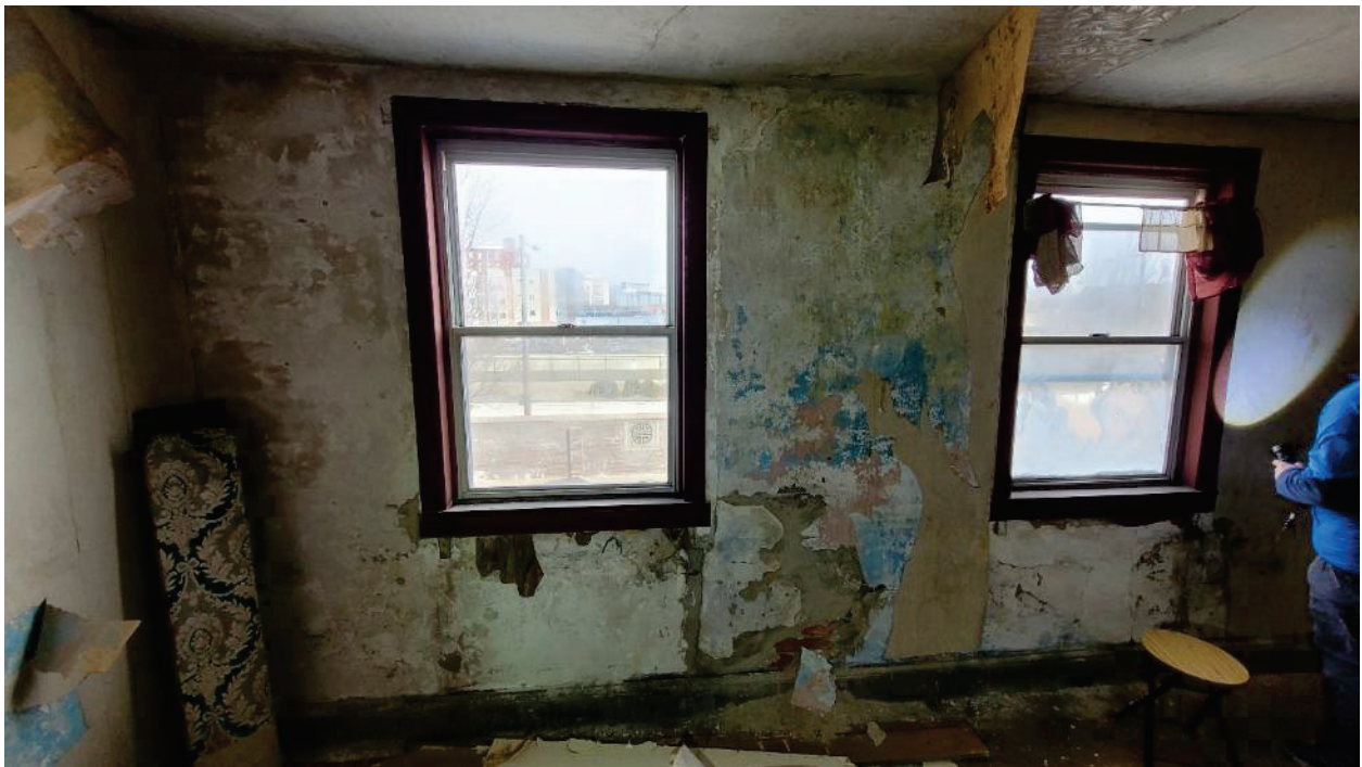
Photo No. 17. View of the interior of the 2 nd floor front wall
