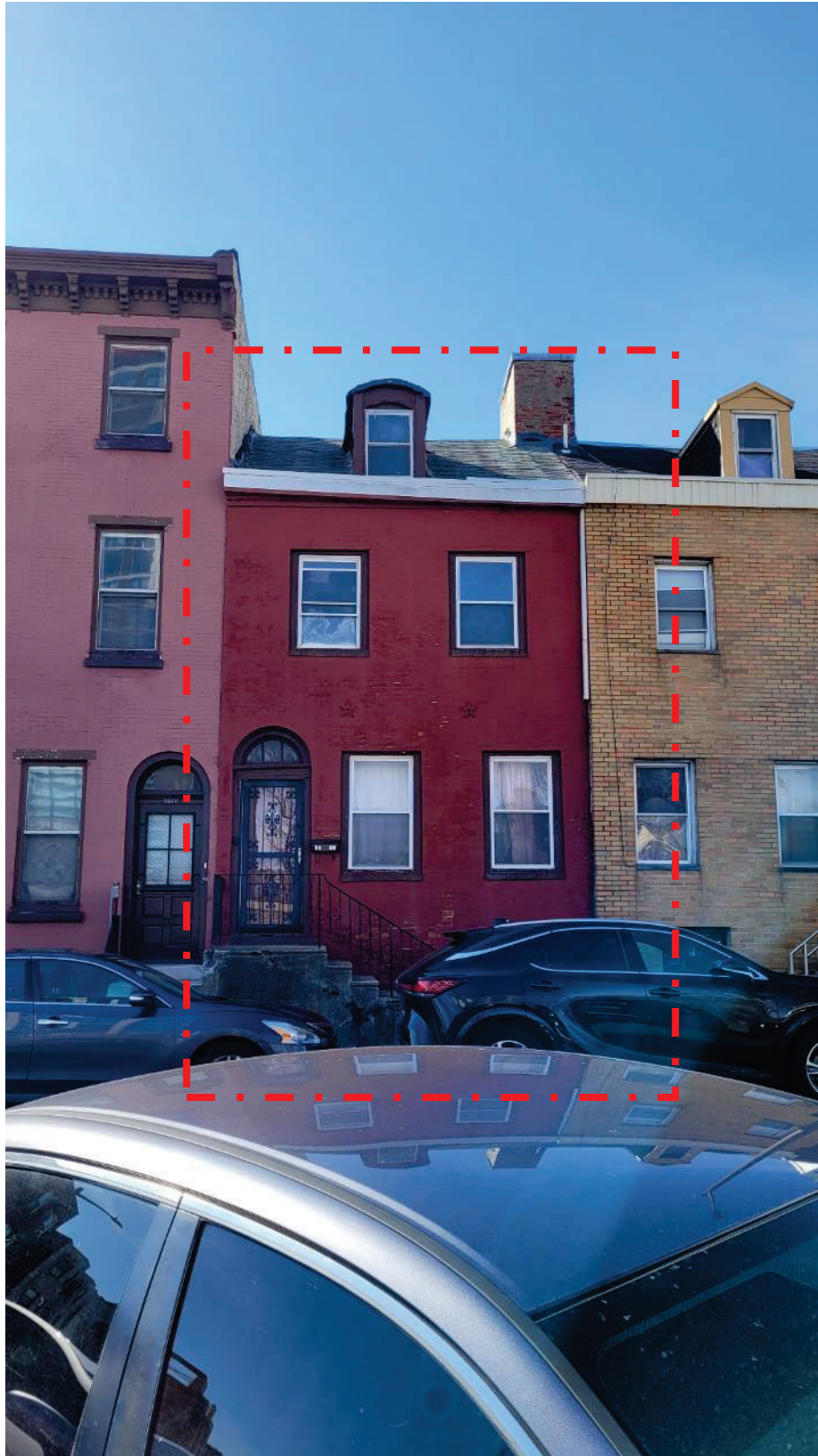
Photo No. 1. Front view of 1018 Winter Street, Philadelphia, PA 19107
