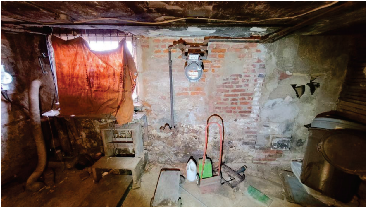
Photo No. 19. View of the front foundation wall
