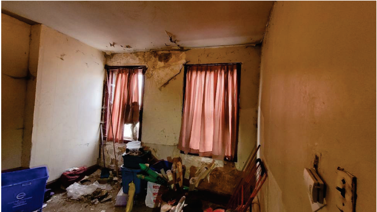
Photo No. 12. View of the interior of the 1 st floor front wall
