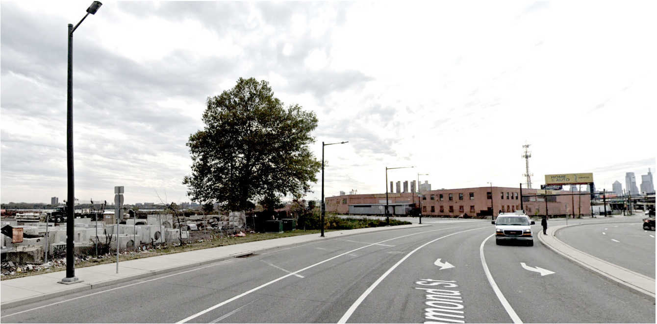
VIEW LOOKING SW FROM RICHMOND
