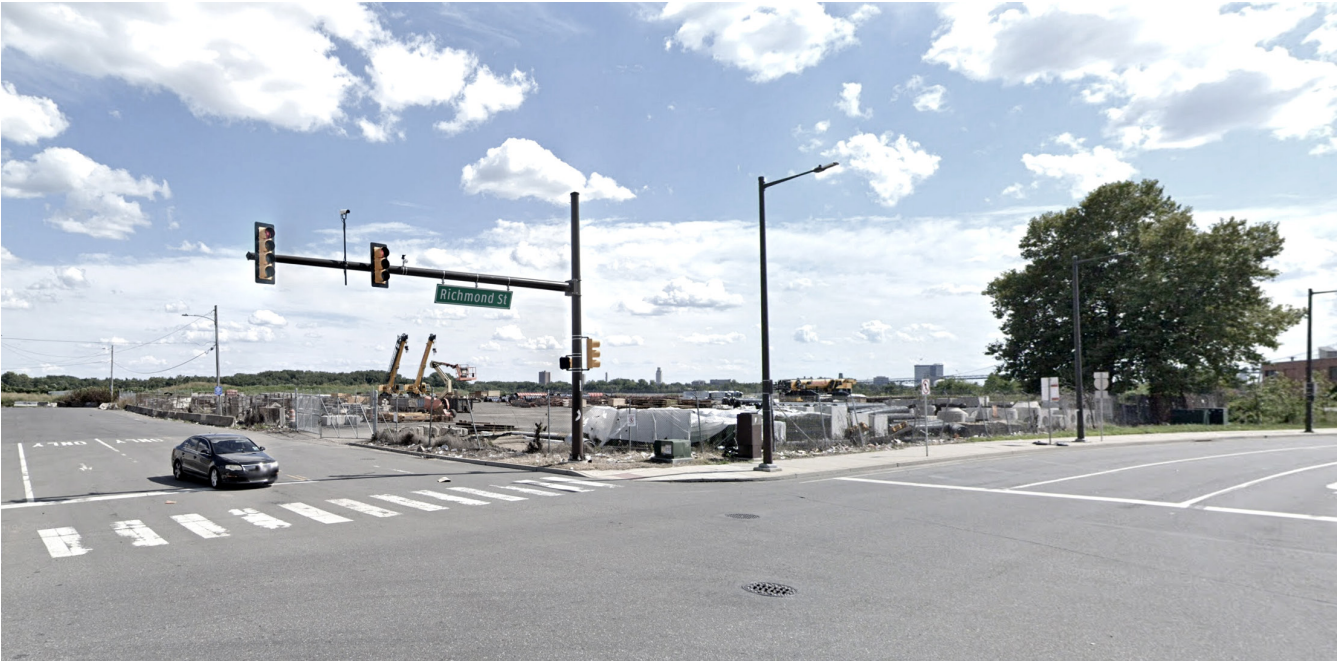
VIEW LOOKING S AT SCHIRRA + RICHMOND
